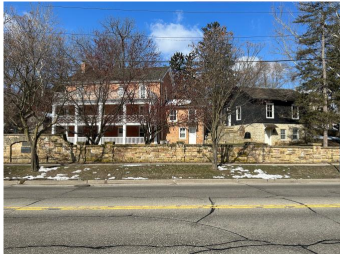
Nakoma Road Tavern View with Exposed Basement
