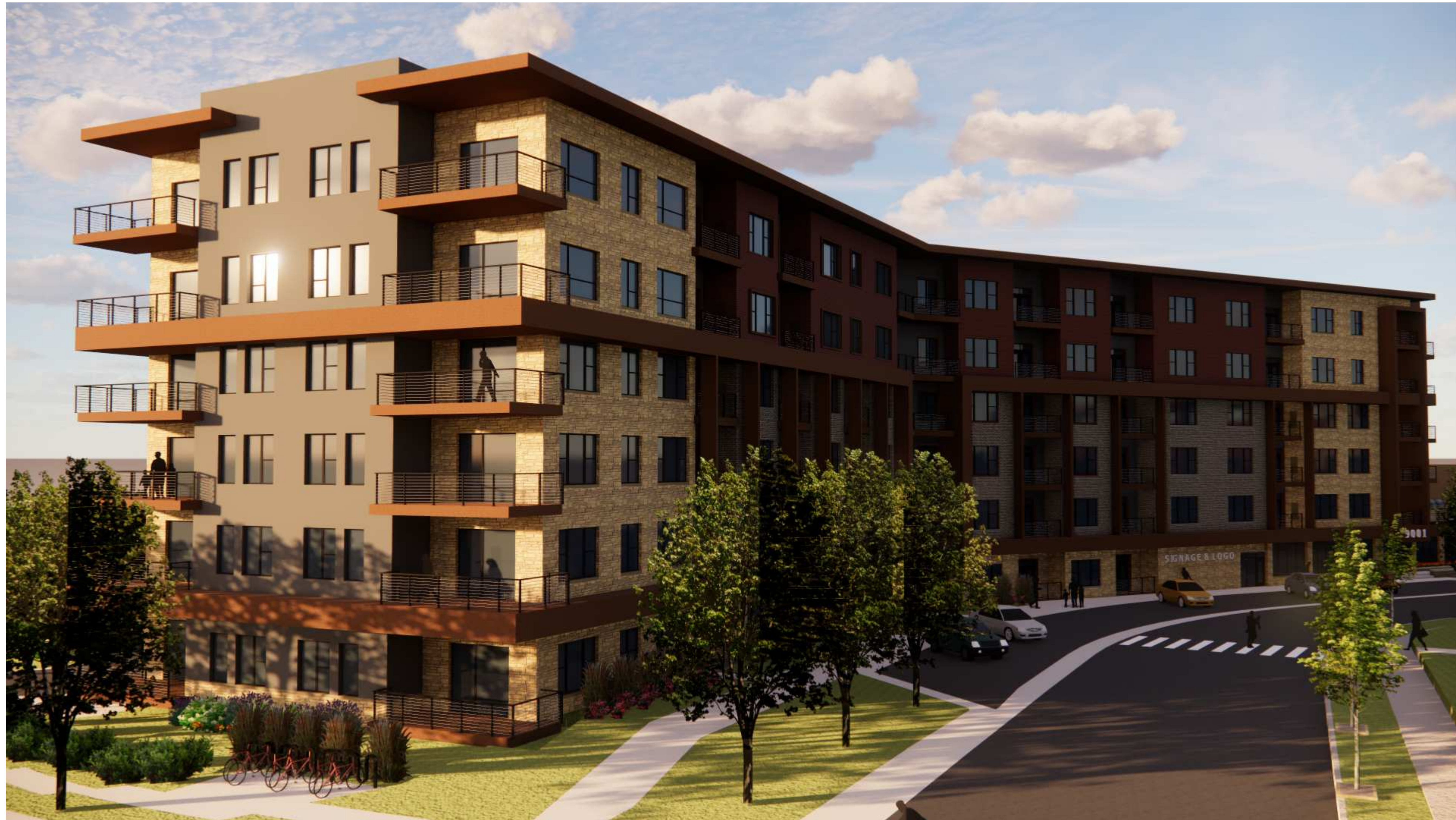
VIEW FROM GEMINI DRIVE & SHARPSBURG DRIVE
