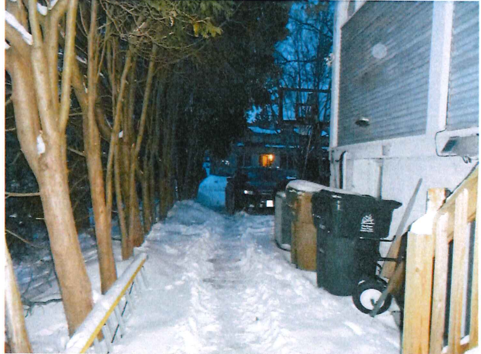
Picture Construction Access looking North
