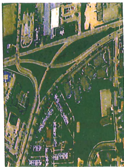
Image 6: Bird's eye view of the Northport Drive - Packers Avenue - Highway CV intersection.
