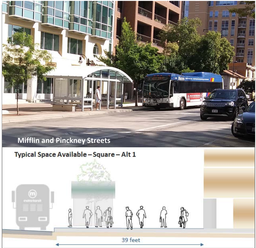
Figure 4-9 Mifflin and Pinckney Bus Stop
