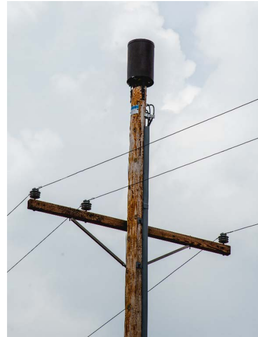
Small cell antenna
