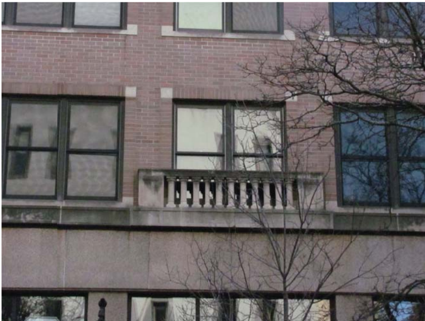
Figure 2. Only a limestone belt course and balustrade at the third floor remain from the original State Street facade.
