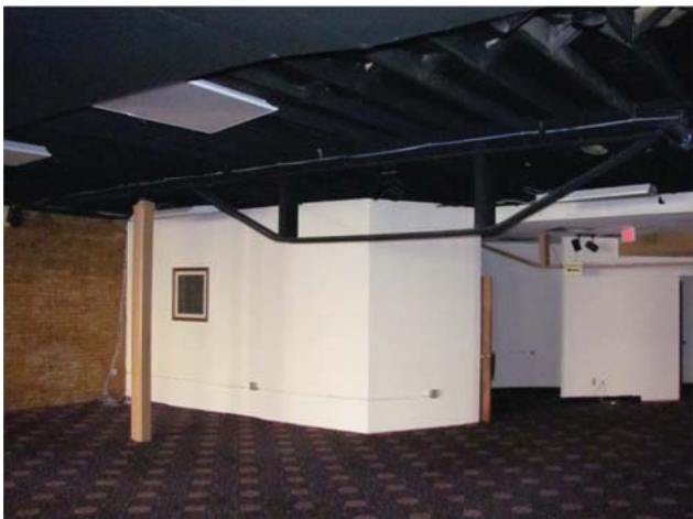
Figure 12. At the third and fourth floors of the building, unique original wood and iron trusses are exposed to view.
