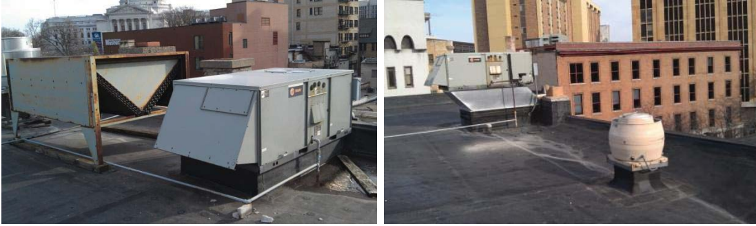
Existing rooftop equipment
