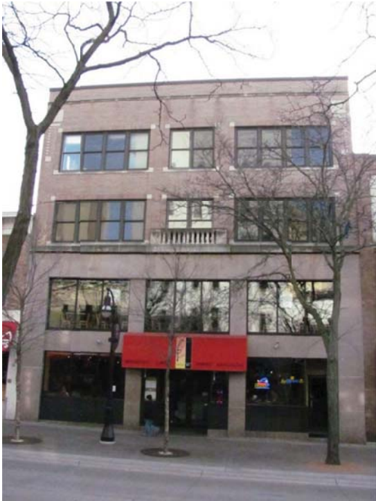
Figure 1. The State Street facade.
