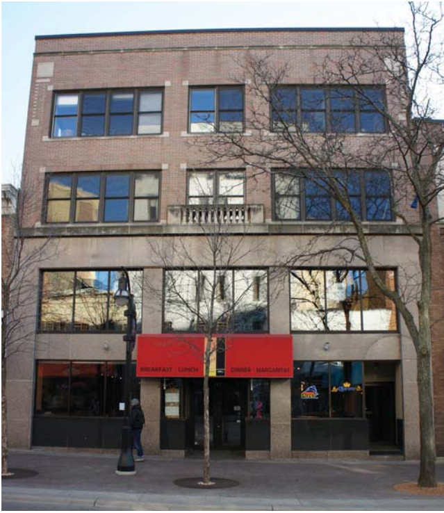
View of Front Facade
