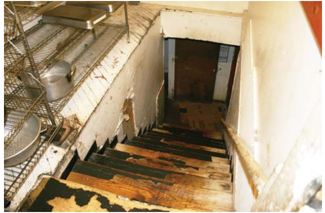
First Floor: View of access to basement
