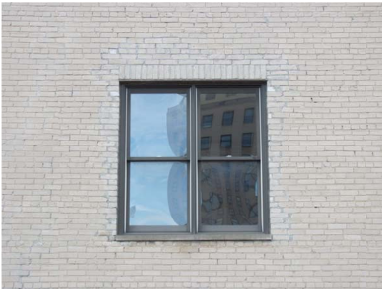
Figure 9. Typical aluminum-clad wood windows.
