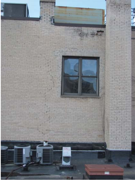
Figure 7. Left. Vertical cracking and localized damage in the brick masonry party wall, which is visible where it extends above the roofs of the adjacent buildings.
