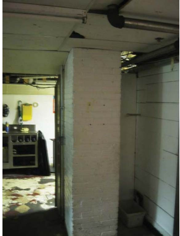
Photo 5 – Basement level brick pier
