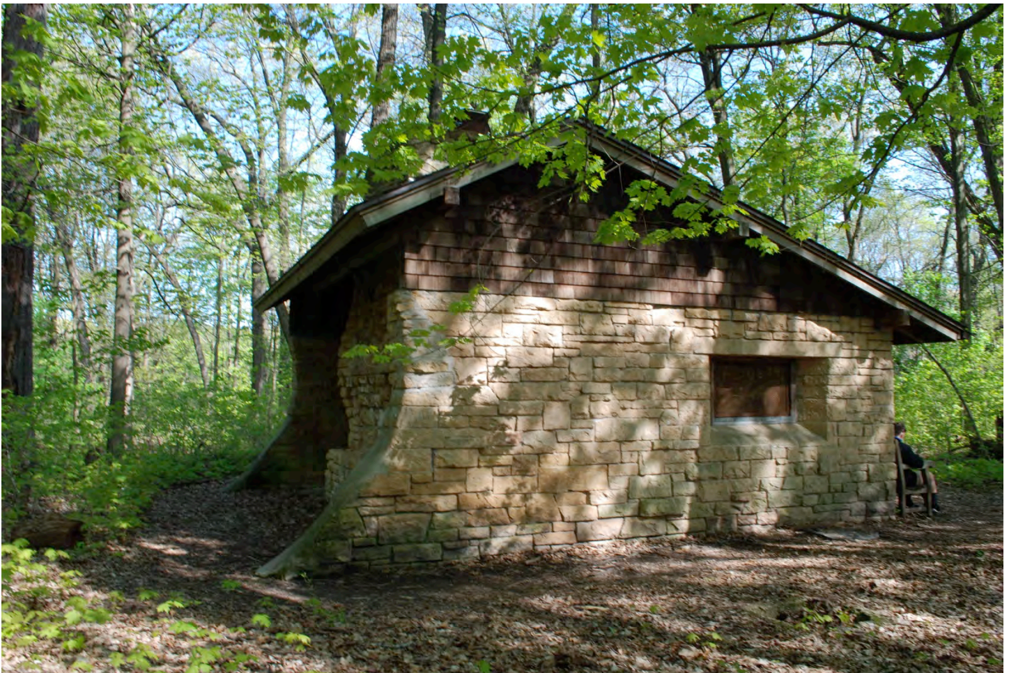
WI_DaneCounty_University of Wisconsin Arboretum_0023 Gallistel Woods Shelter, camera facing southeast.
