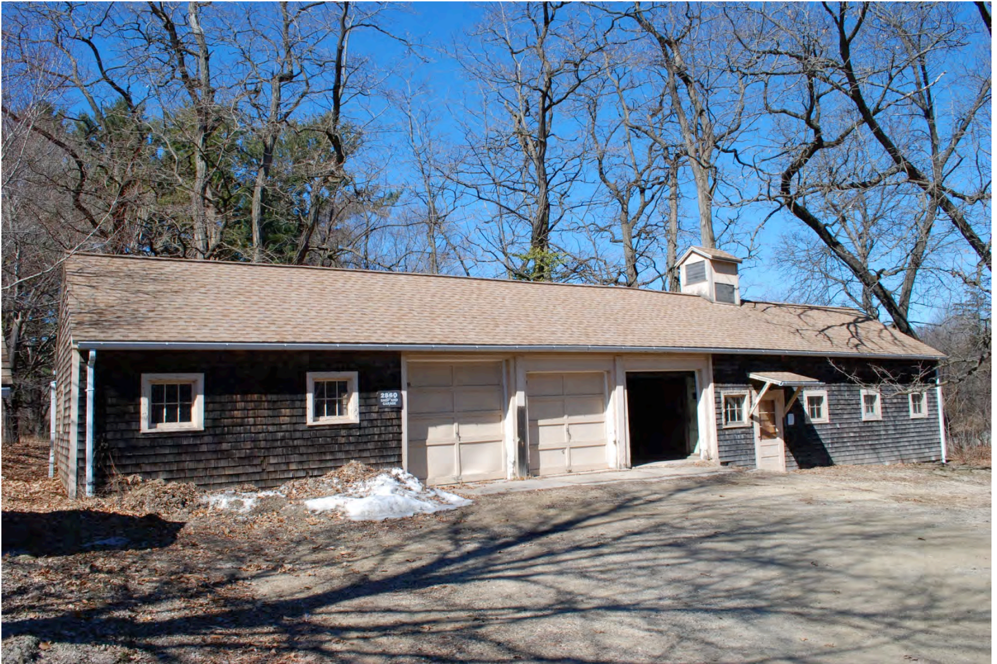
WI_DaneCounty_University of Wisconsin Arboretum_0012 Carpentry Workshop and Warehouse, camera facing west.
