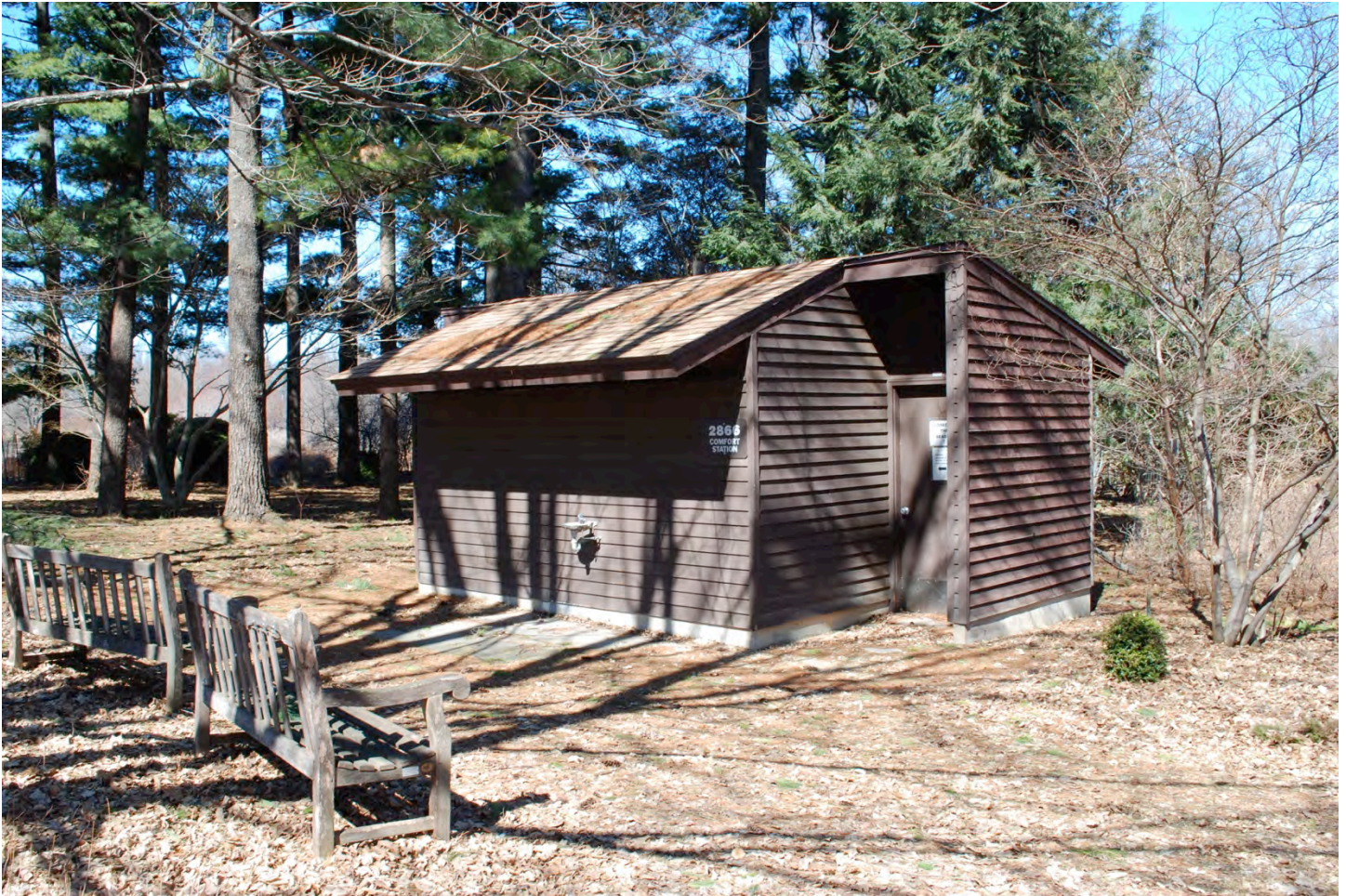
WI_DaneCounty_University of Wisconsin Arboretum_0016 Comfort Station, camera facing northwest.
