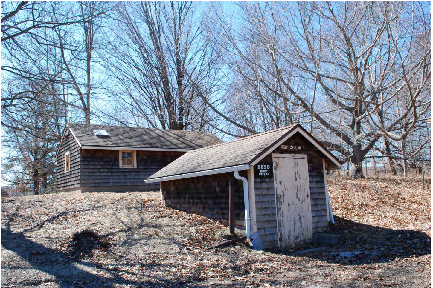
WI_DaneCounty_University of Wisconsin Arboretum_0014 Root Cellar and Main Pumphouse, camera facing westerly.
