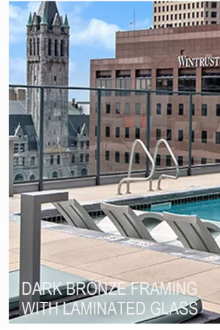
GLASS GUARDRAIL ASSEMBLY
