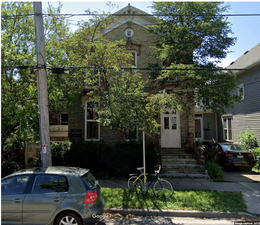
West Adjacent Neighbor (Kircher House)
