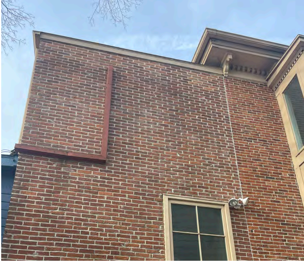
East Elevation of Late-Brick Addition
