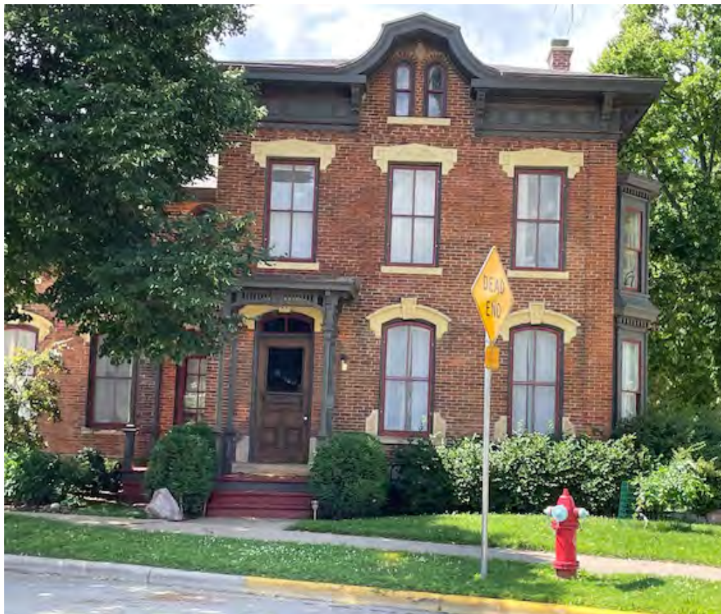
Ott House (north-east kitty-corner of residence)
