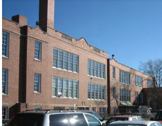
A. 210 S. Brooks St. View looking southeast on Mound St.
