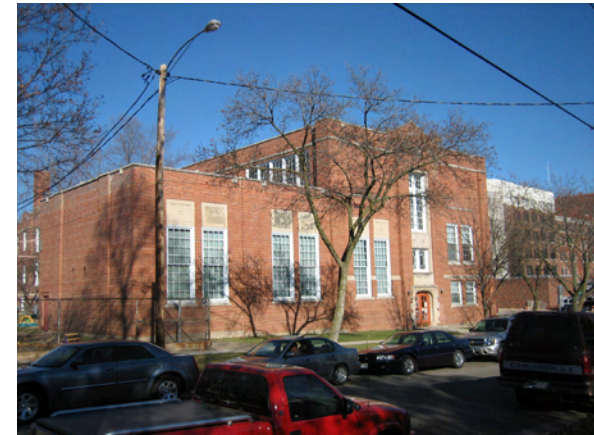
A. 210 S. Brooks St. View looking north on Chandler St.
