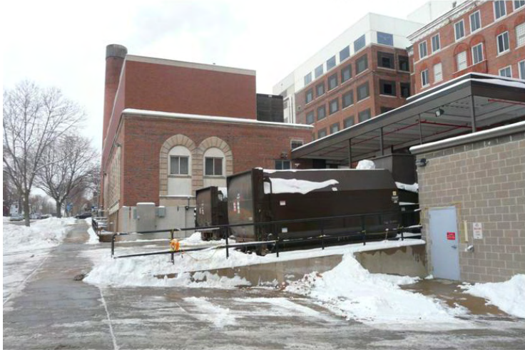
Figure 02: Photo of Existing Loading Area
