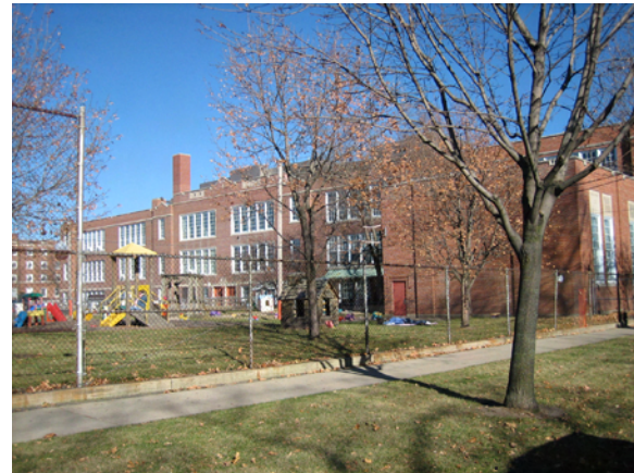
A. 210 S. Brooks St. View looking east on Chandler St.
