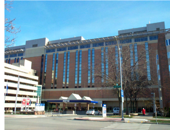
B. 202 S. Park St. View looking east at main entrance from Brooks St.
