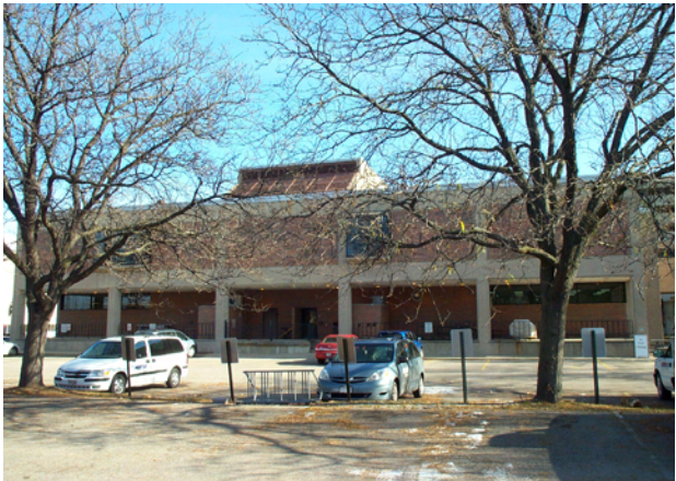
A. 1011 Milton St. View of east elevation.
