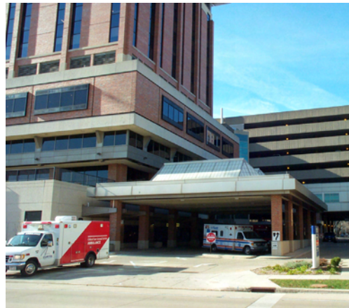
H. 202 S. Park St. View of emergency entrance from Park St.
