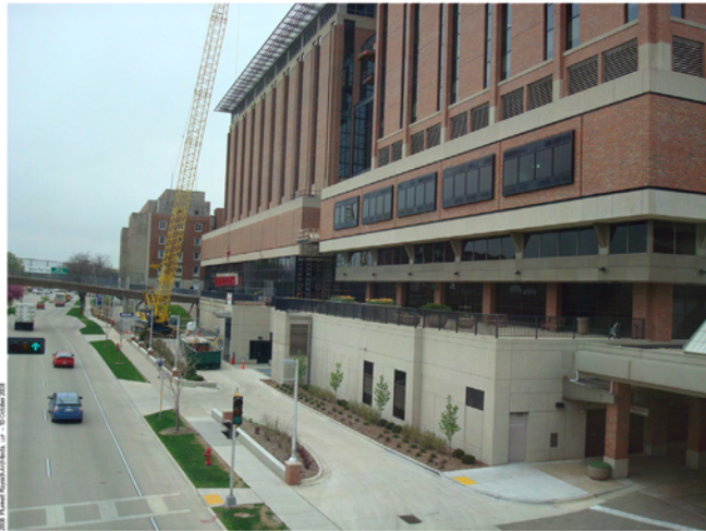
Existing View from Park Street - Looking South
