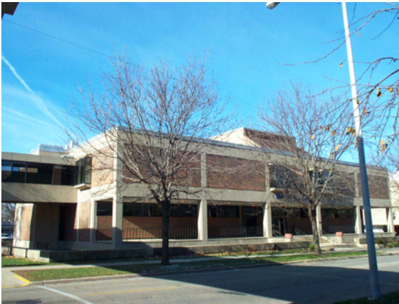
A. 1011 Milton St. View of south and west elevations from Brooks St..
