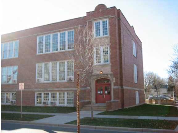
A. 210 S. Brooks St. View looking west on Brooks St.
