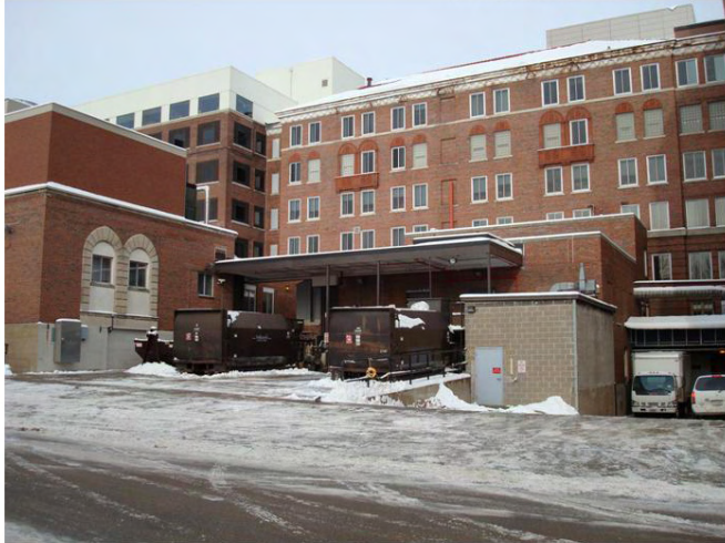
Figure 01: Photo of Existing Loading Area
