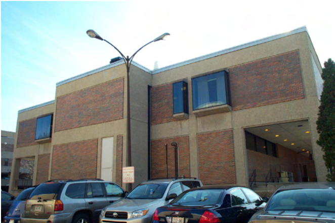
A. 1011 Milton St. View of north elevation.
