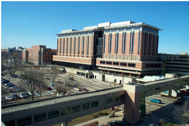
G. 202 S. Park St. View of east elevation from across Park St.
