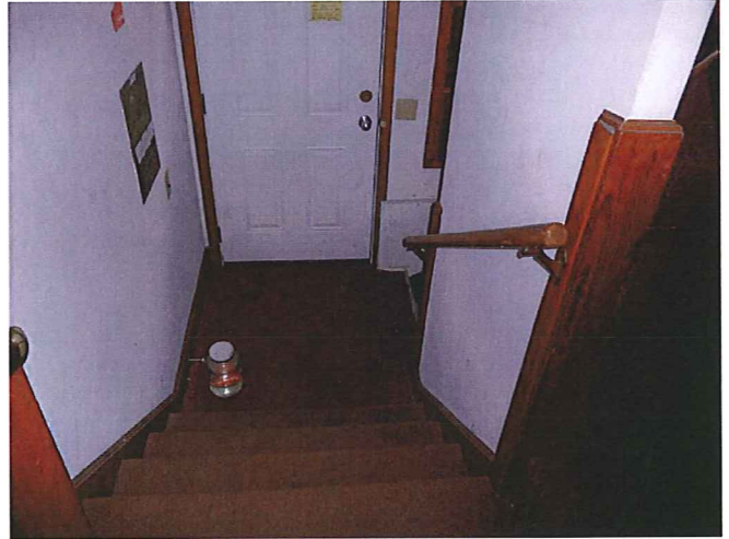
BUILDING ENTRY AND COMMON STAIR
