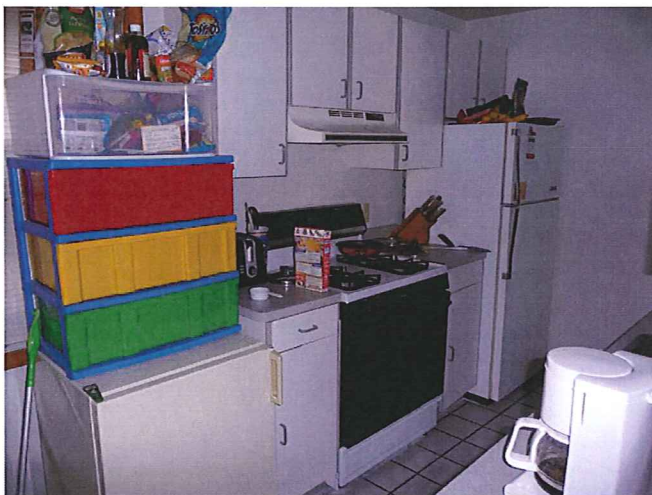
TYPICAL UNIT KITCHEN
