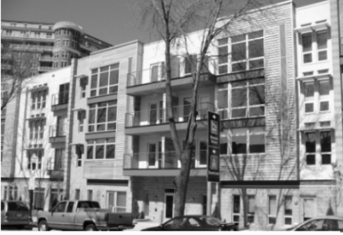
Figure D3: Facade Modulation
