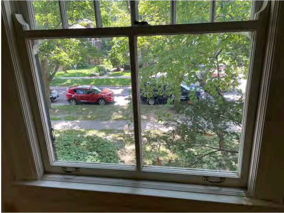
Double-hung windows on main & upper levels
