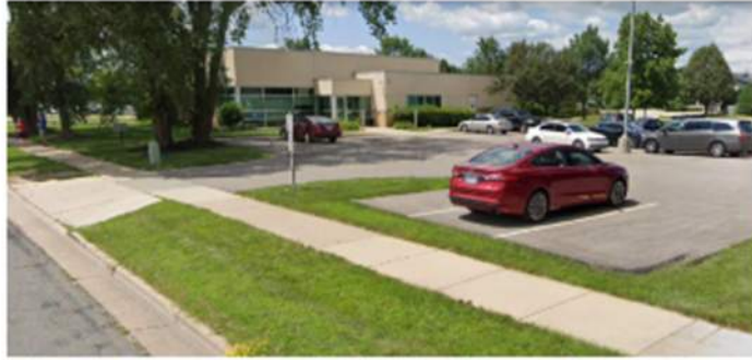
NORTH STOUGHTON HEALTH CENTER
