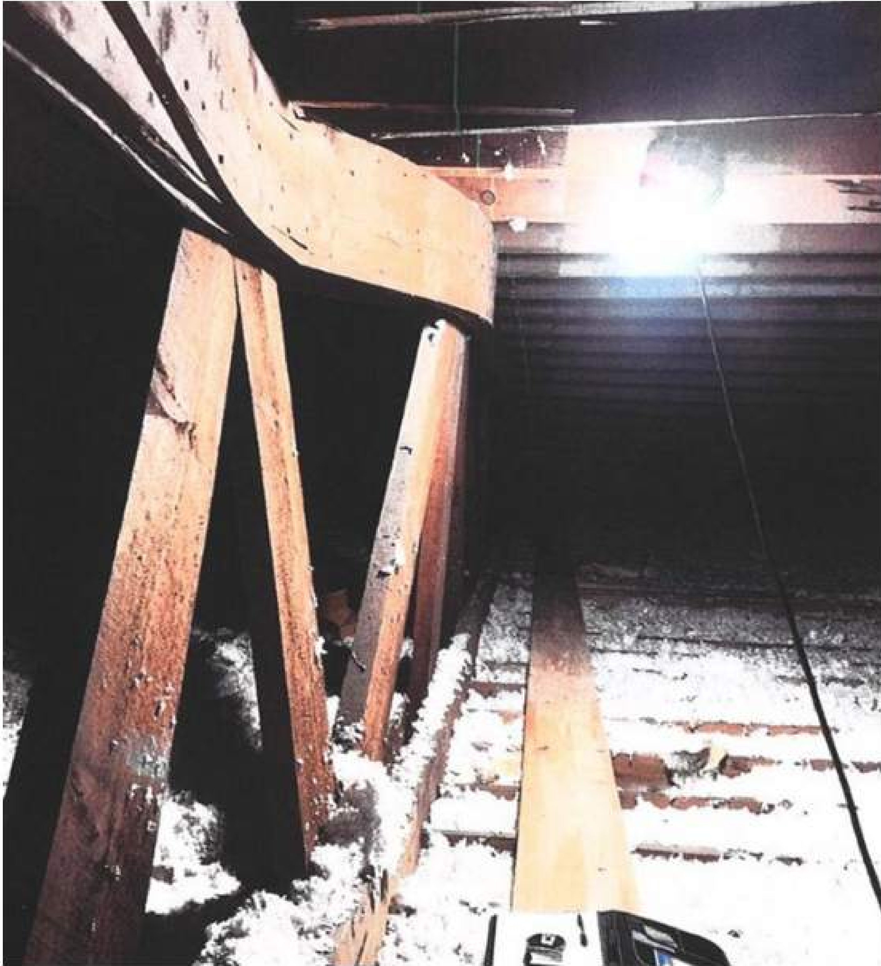
ROOF TRUSS FAILURE
