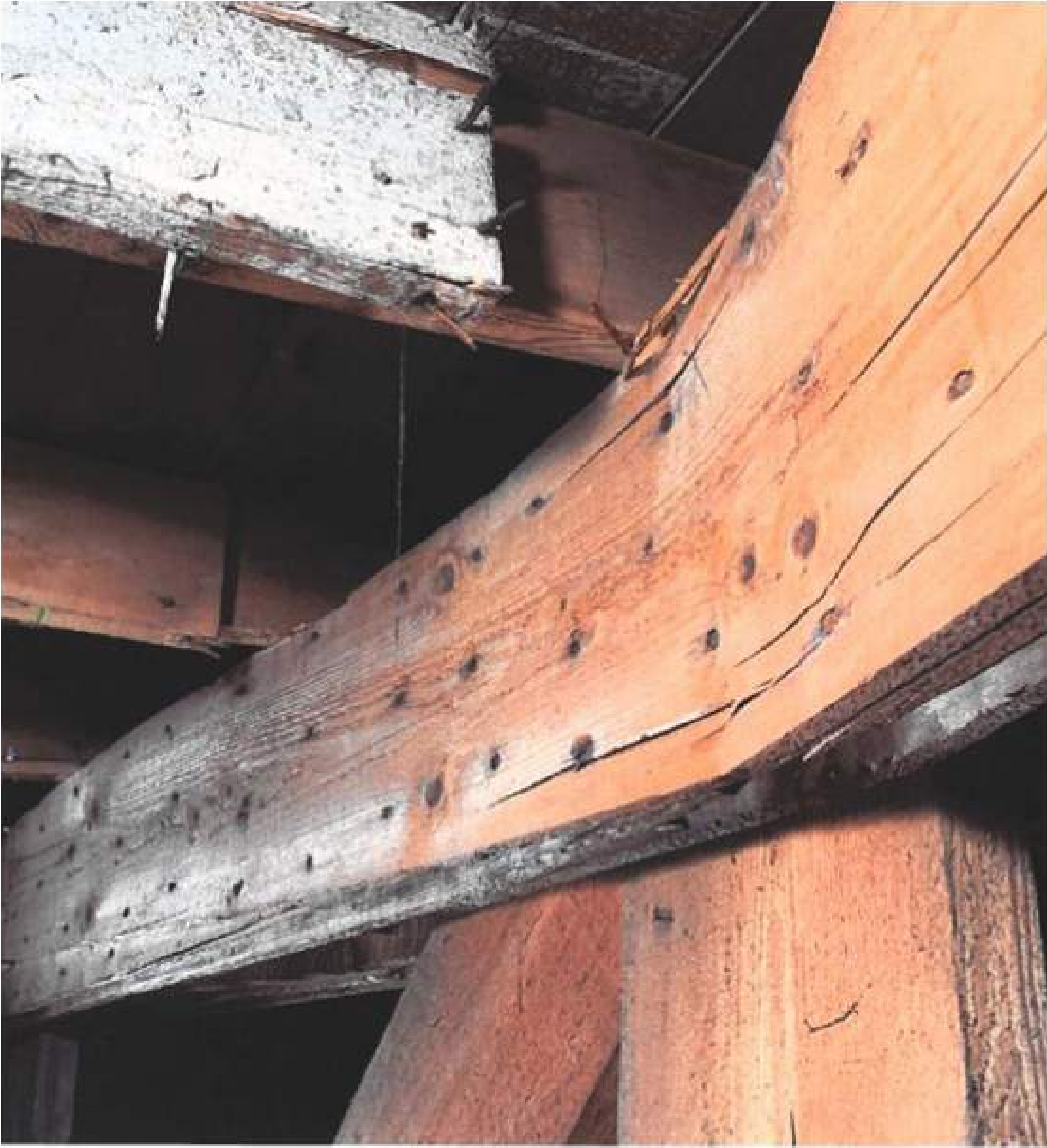
ROOF TRUSS & PURLIN FAILURE
