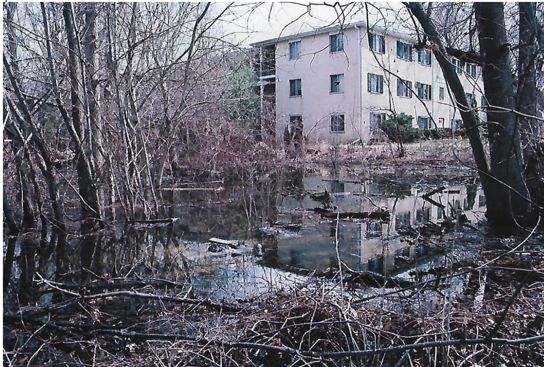
View of 222 Merry from 220 Merry during flooding, 2018 flooding was far worse.
