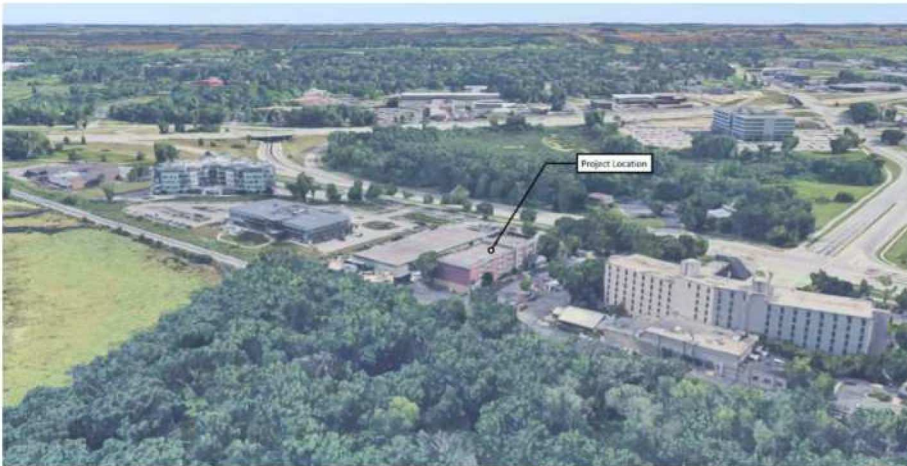
AERIAL VIEW OF SITE LOOKING SOUTH
