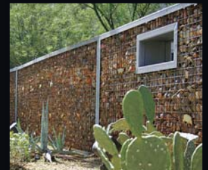
Rock Wall Fencing
