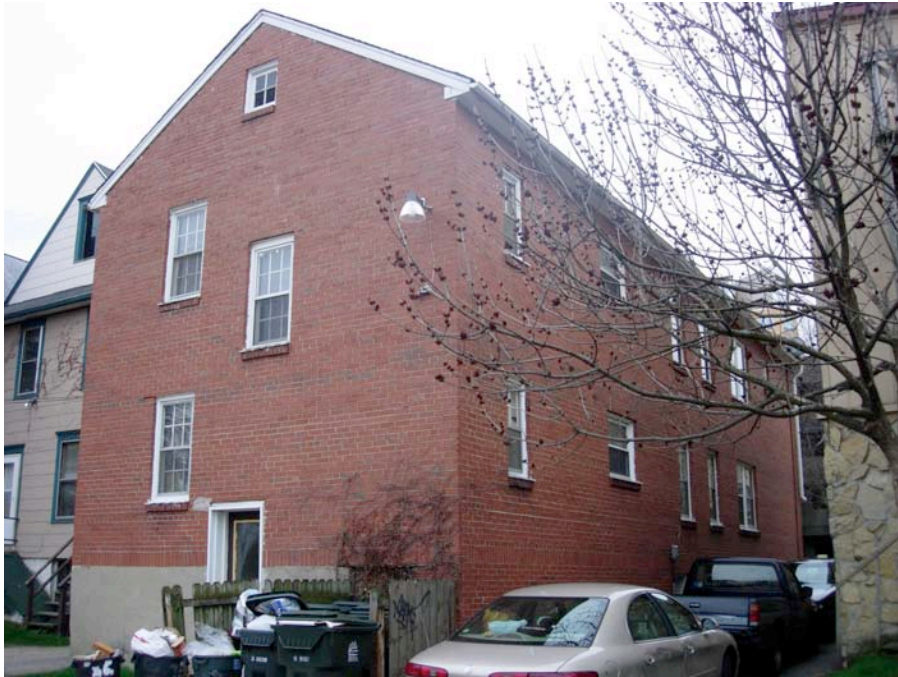
View from North East
