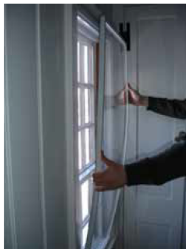
Interior storm panel.
