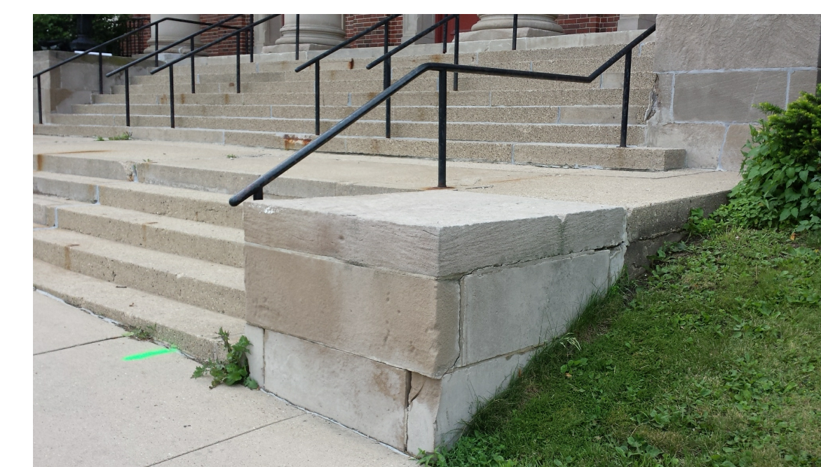
1609 UNIVERSITY AVE. - STAIR PLINTHS AND HANDRAILS
