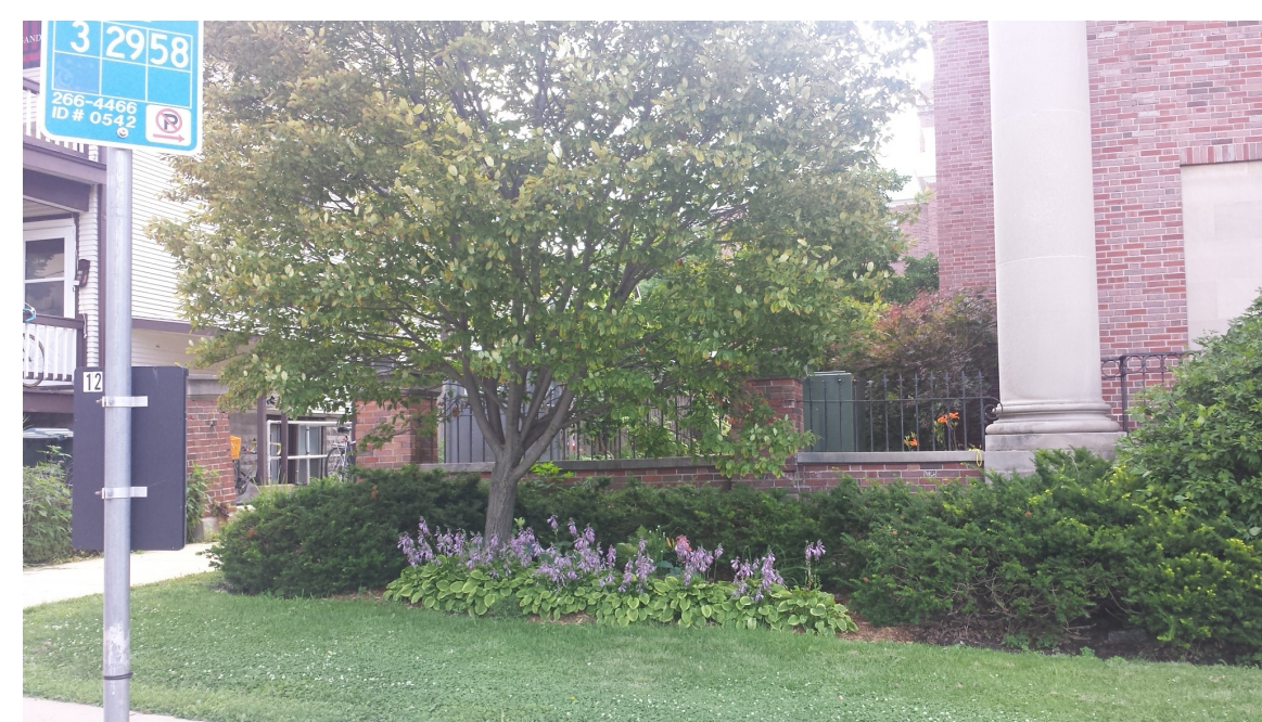
1609 UNIVERSITY AVE. - EXISTING BRICK WALL
