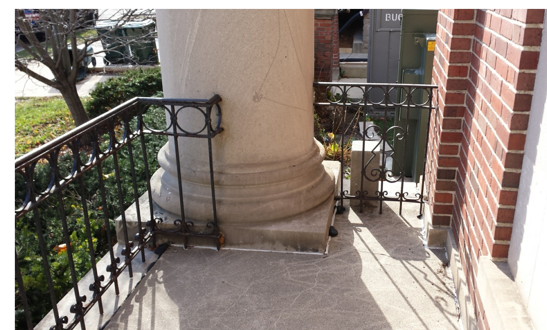
1609 UNIVERSITY AVE. - EXISTING STEEL RAILING
