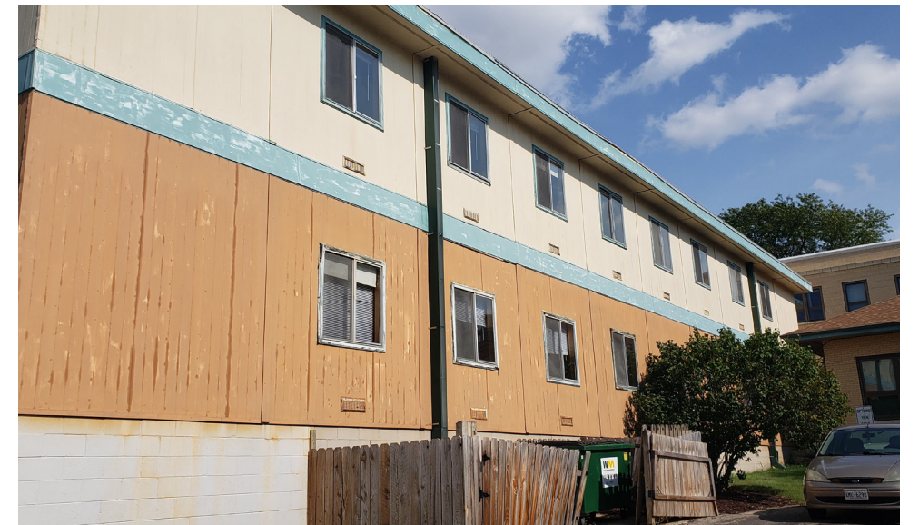
22 N. Second St. Building Exteriors Site Demolition Images
