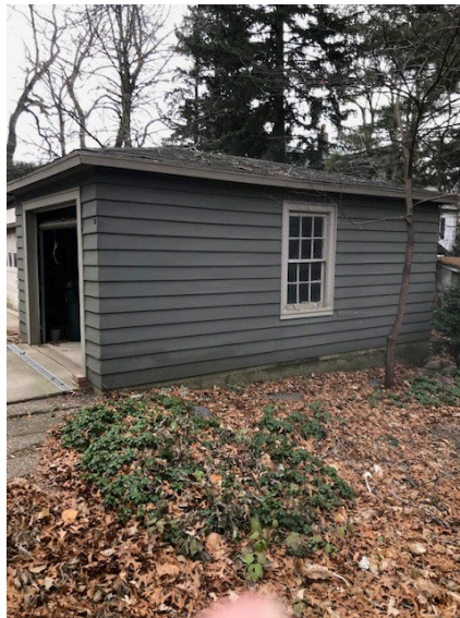
SIDE OF EXISTING GARAGE
