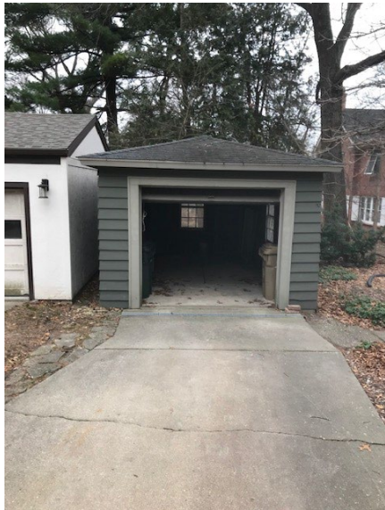
FRONT OF EXISTING GARAGE
