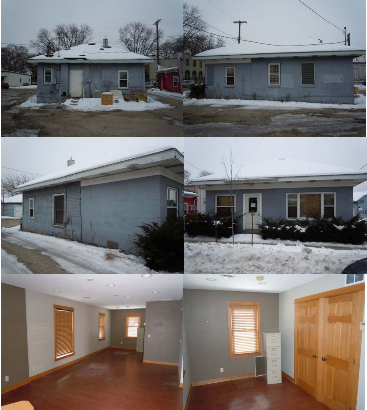
212 S. Baldwin Street Structure
