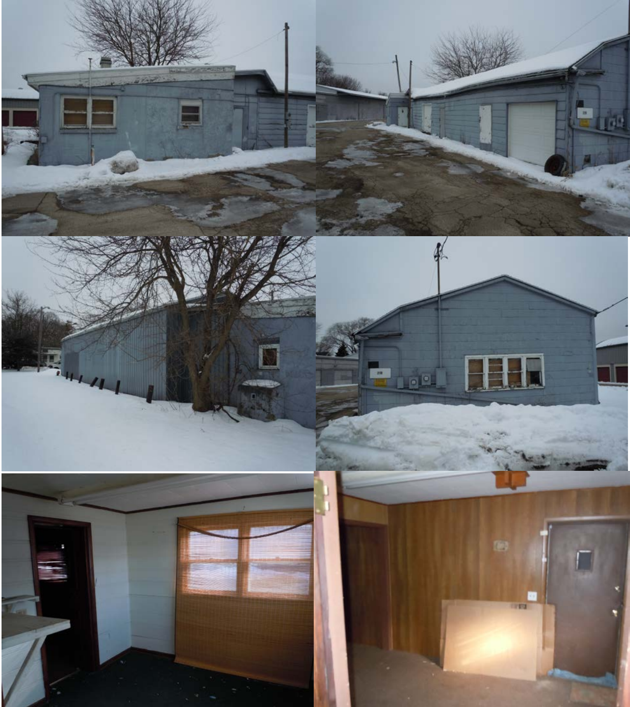
210 S. Baldwin Street Structure
