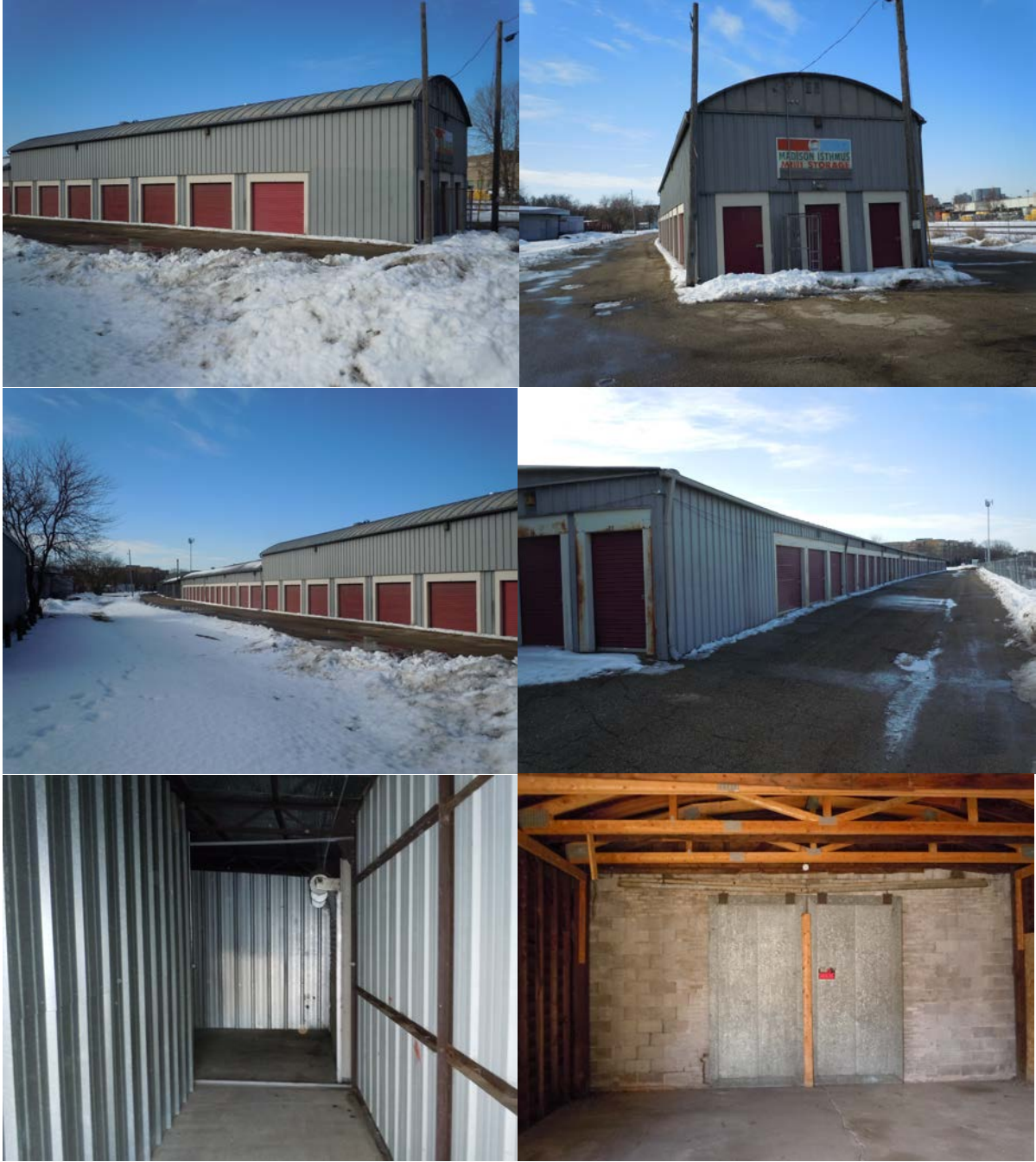
202-208 S. Baldwin Street Structure
