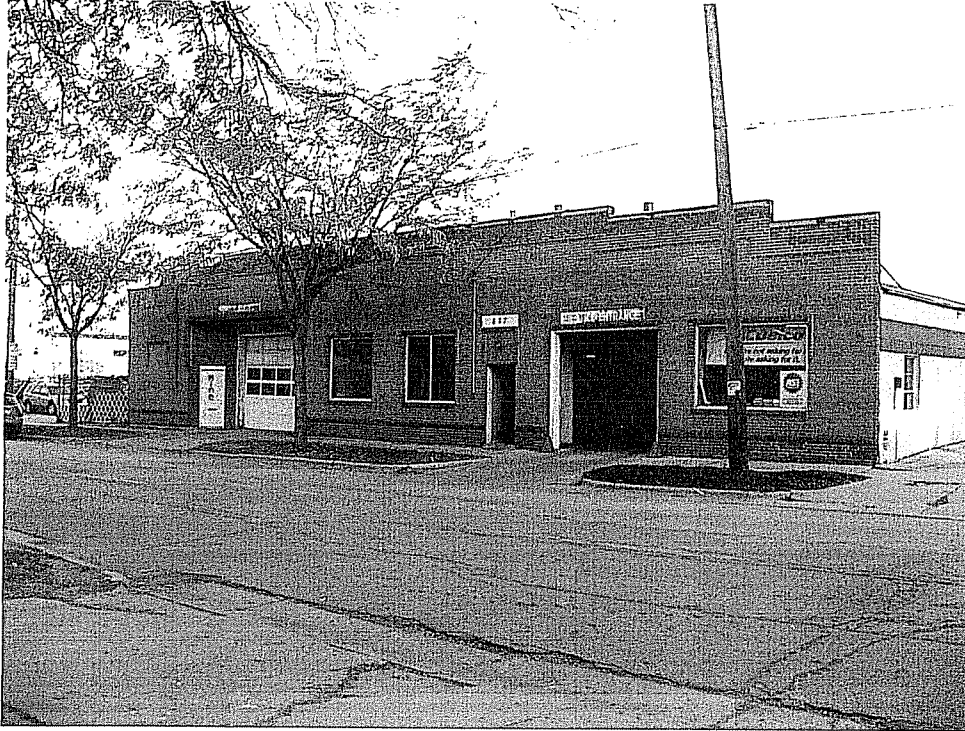
Existing Building to be Demolitioned
