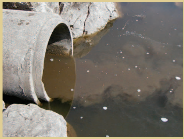
Polluted stormwater from neighborhood streets and other storm drain sources enters Lake Wingra.
