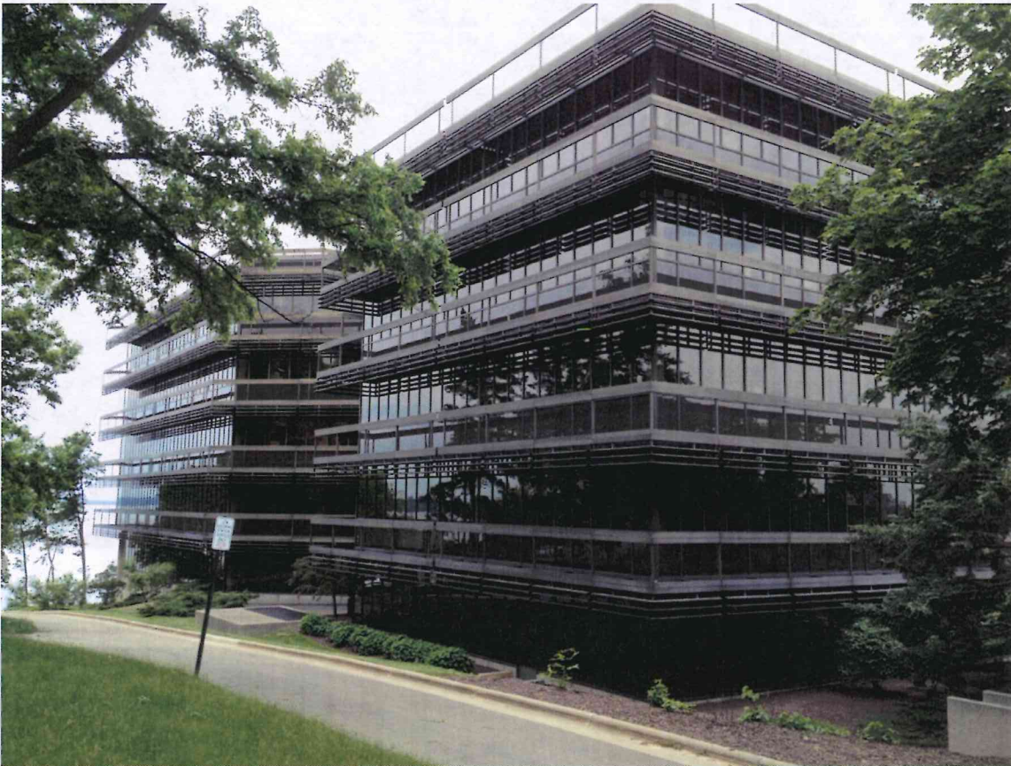
Office building to the north
