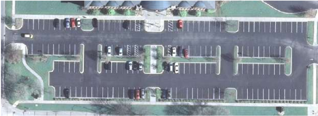
14% Landscaped Coverage within Interior of Parking Lot
