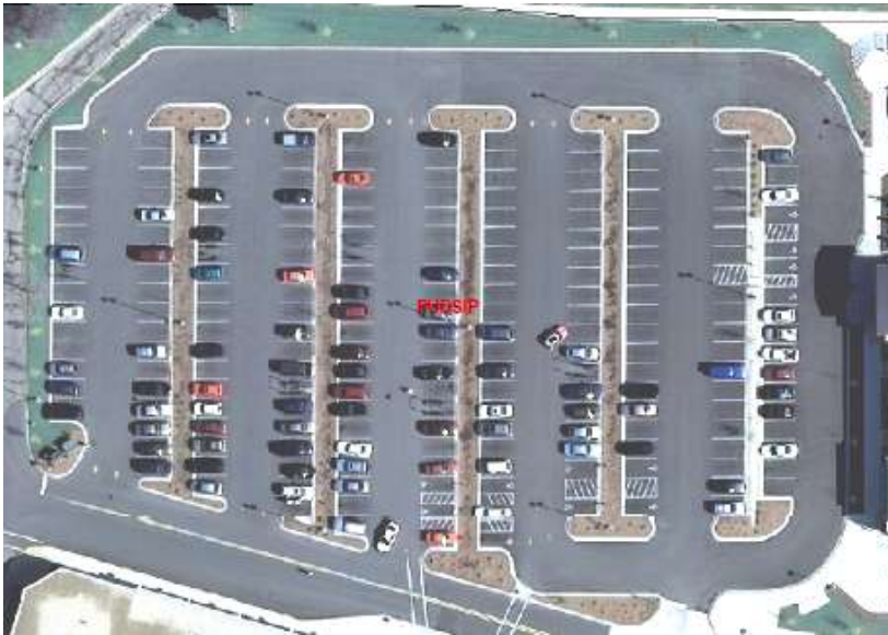
12% Landscaped Coverage within Interior of Parking Lot
