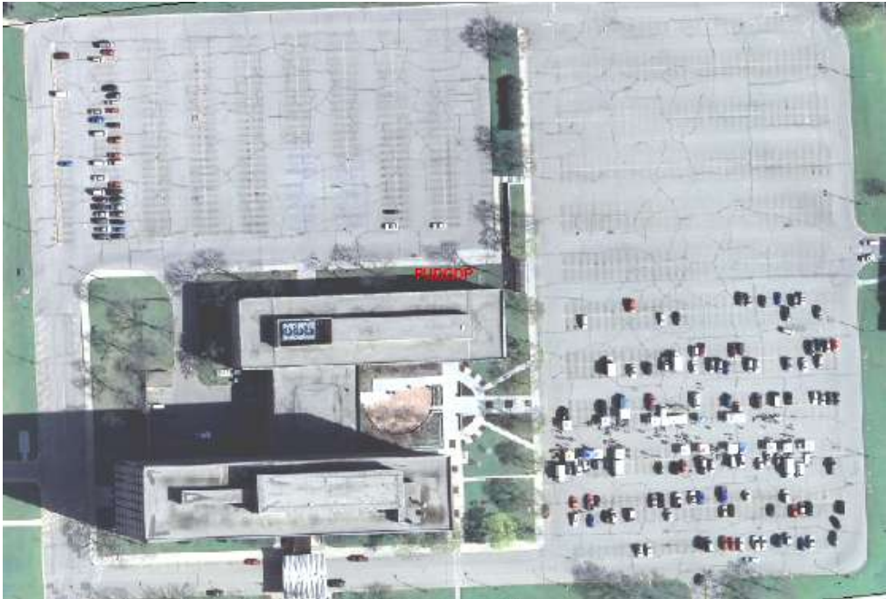
1% Landscaped Coverage within Interior of Parking Lot
