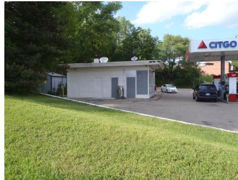
ADJACENT GAS STATION TO EAST
