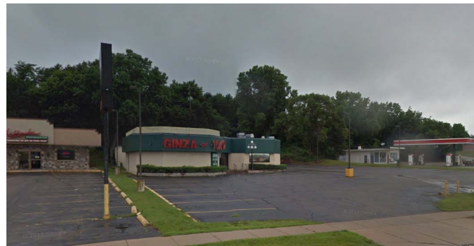
BOTH ADJACENT BUILDINGS
