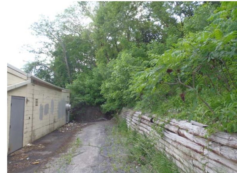
VIEW OF REAR OF BUILDING
