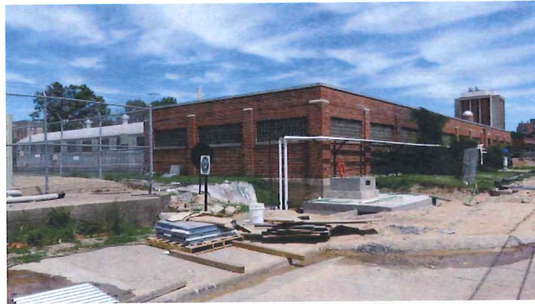
View 11: Southwest corner of building (current utility work in progress)
