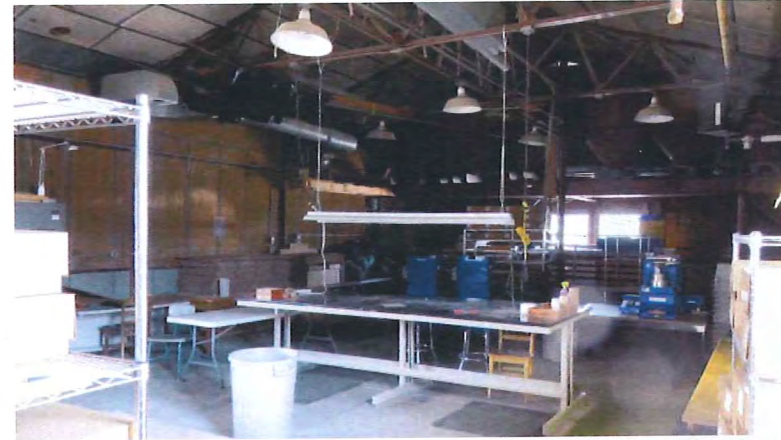
View 17: Room E2, view north
