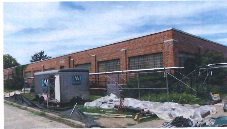
View 14: Southeast corner of building (current utility work in progress)
