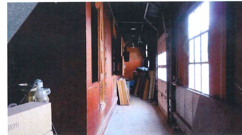
View 35: Room C3, view north
