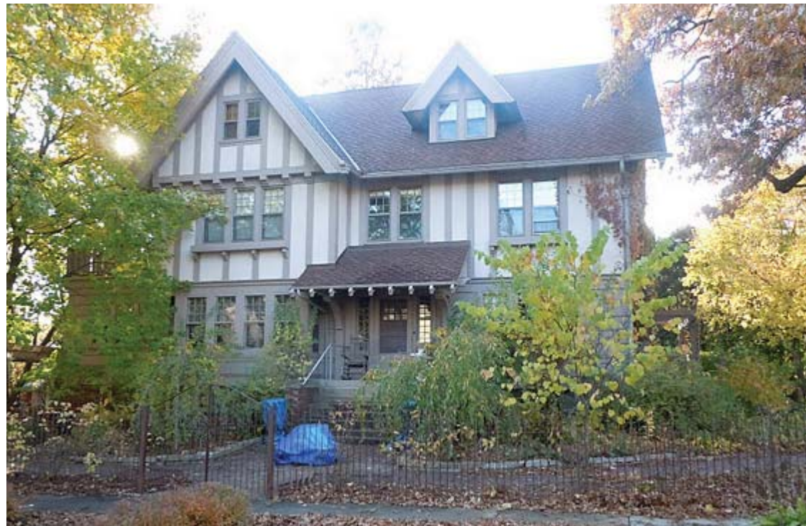
N: 14 North Prospect Roof: High Gable Facing Street and Side + Flat Roof Addition Facade: Stucco, Vertical Exposed Timbers
