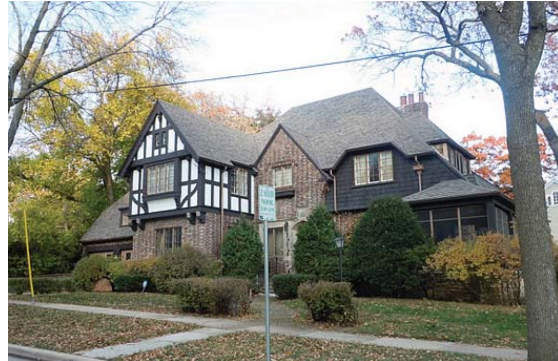
Q: 101 North Prospect Ave Roof: High Hip, Shallow Overhang Facade: Brick, Stucco, Exposed Timbers, Shingles
