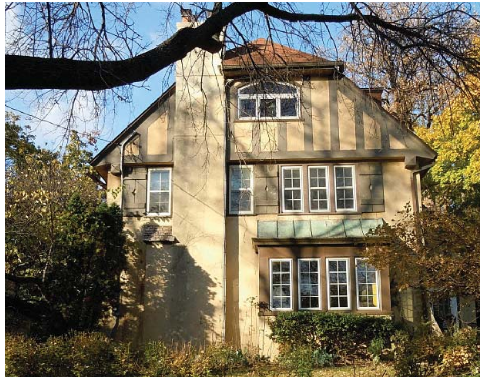
L: 2110 Chadbourne Ave Roof: Gambrel Hip Facing Front Facade: Stucco, Vertical Exposed Timbers
