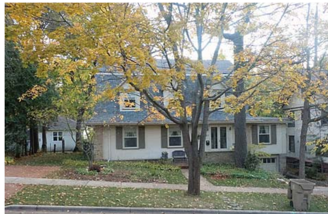
F: 2111 Van Hise Ave Roof: High Gambrel, Facing Side + Garage Flat Roof Facade: Stucco, Stone
