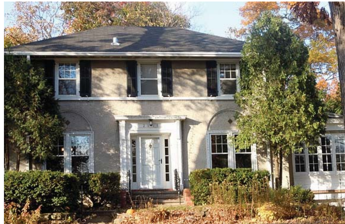
R: 2016 Van Hise Ave Roof: Low Hip + Flat Roof Garage Facade: Stucco
