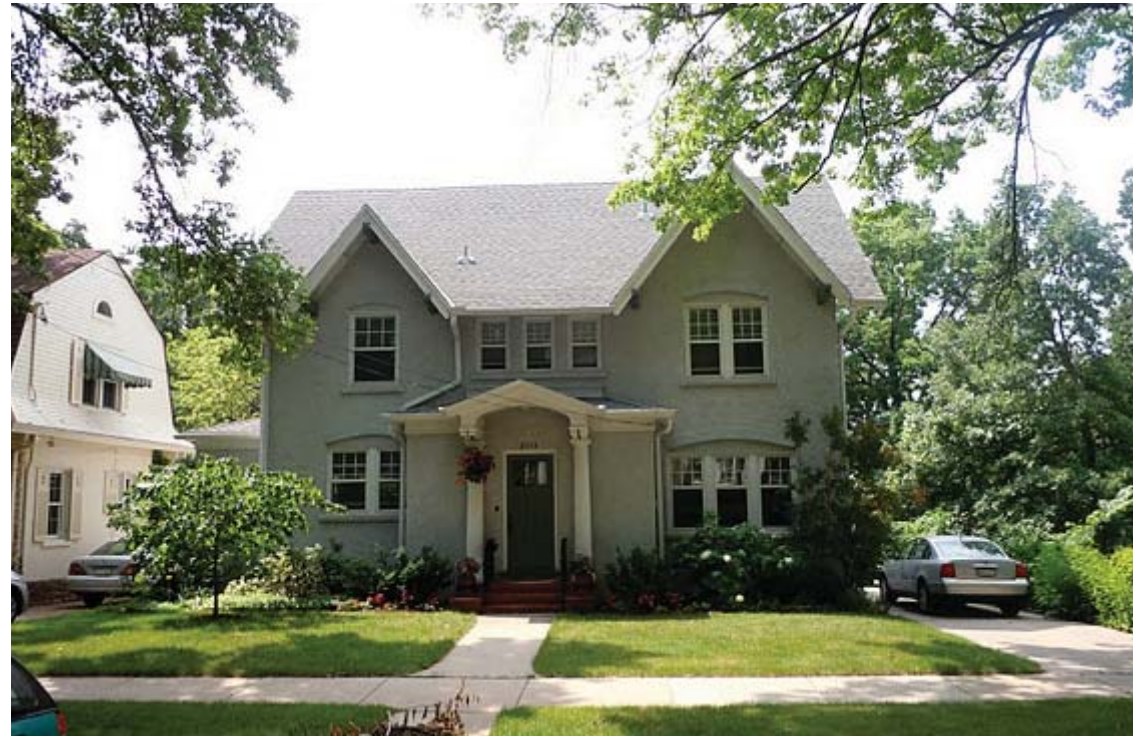
C: 2015 Van Hise Ave Roof: High Gable, Facing Side Facade: Stucco
