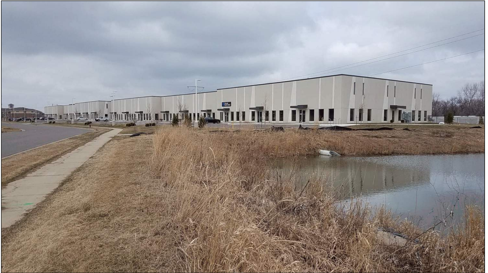
Flex Space Commercial Building 5004-5032 Tradewinds Parkway)
