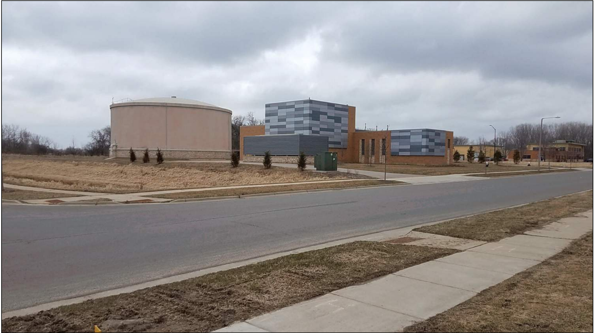
Madison Water Utility Well No. 31 4901 Tradewinds Parkway
