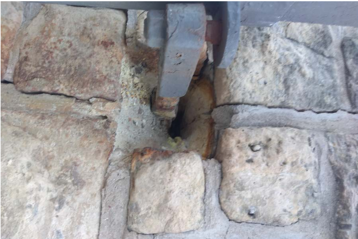
Gate- right side. Close up view of gate mount and crumbling support.
