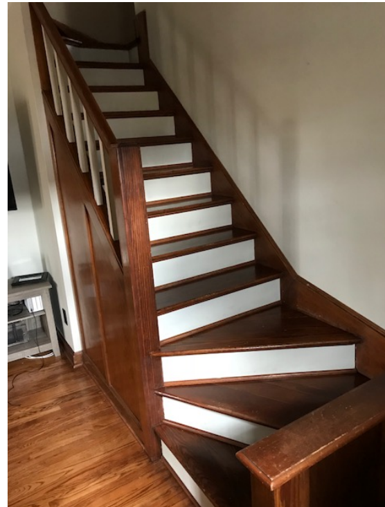
THE WAY IN WHICH THE 1980'S ERA ADDITON WAS ADDED TO THE HOUSE CREATED AN UNSAFE CONDITION AT THE EXISTING WINDER OF THE STAIRCASE
