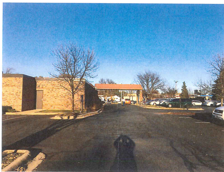
EXISTING CANOPY WITH DRIVE
