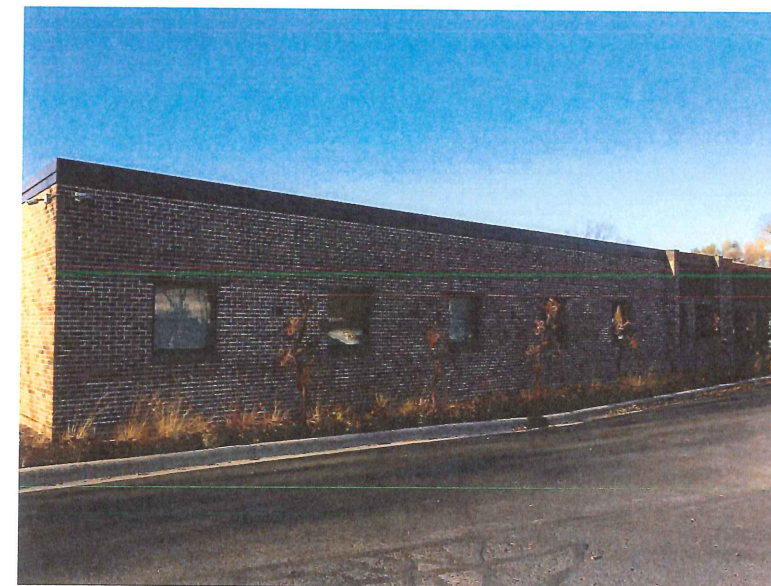
EXISTING SOUTH WALL
