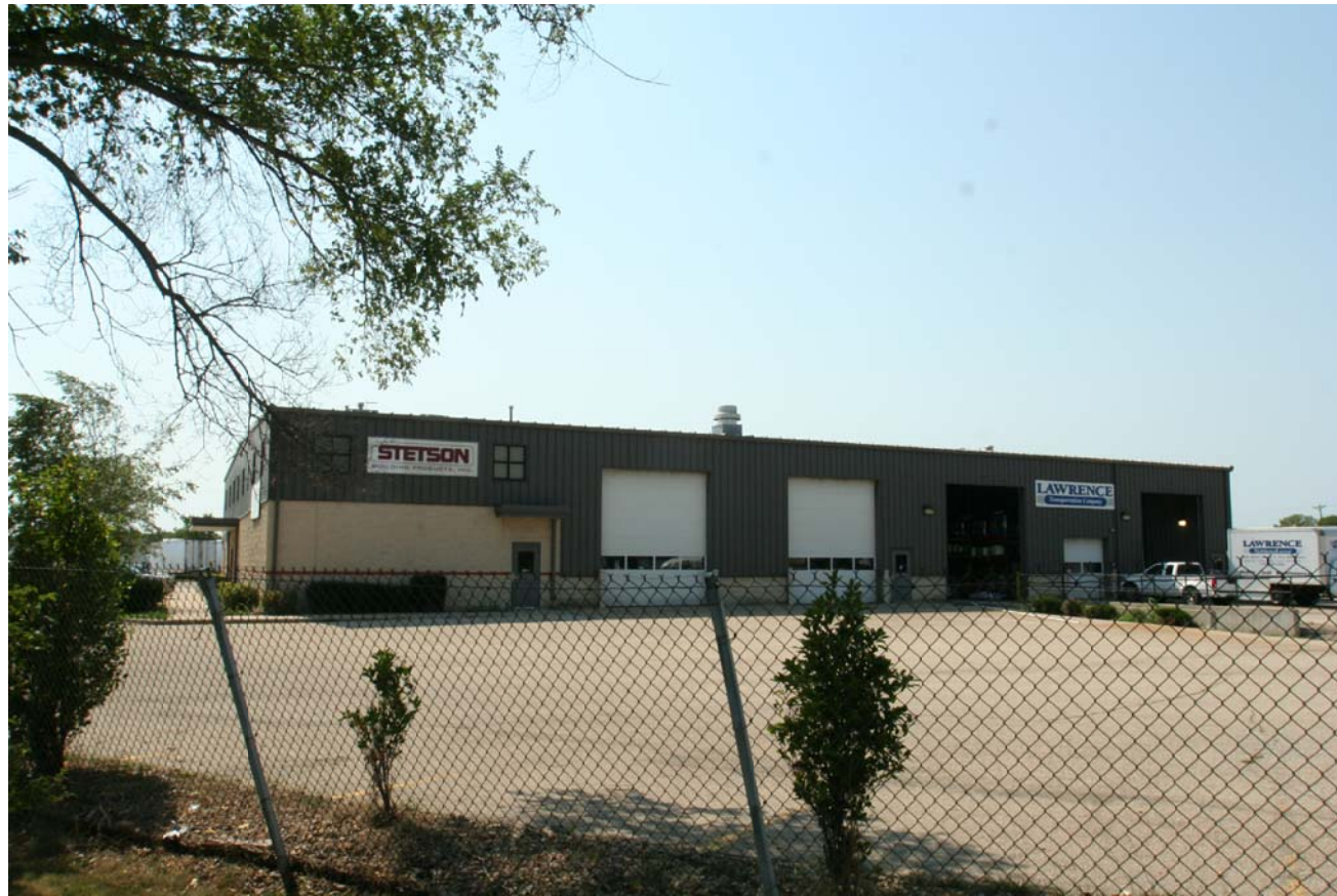
L 4015 TERMINAL DR. - STETSON BUILDING PRODUCTS
