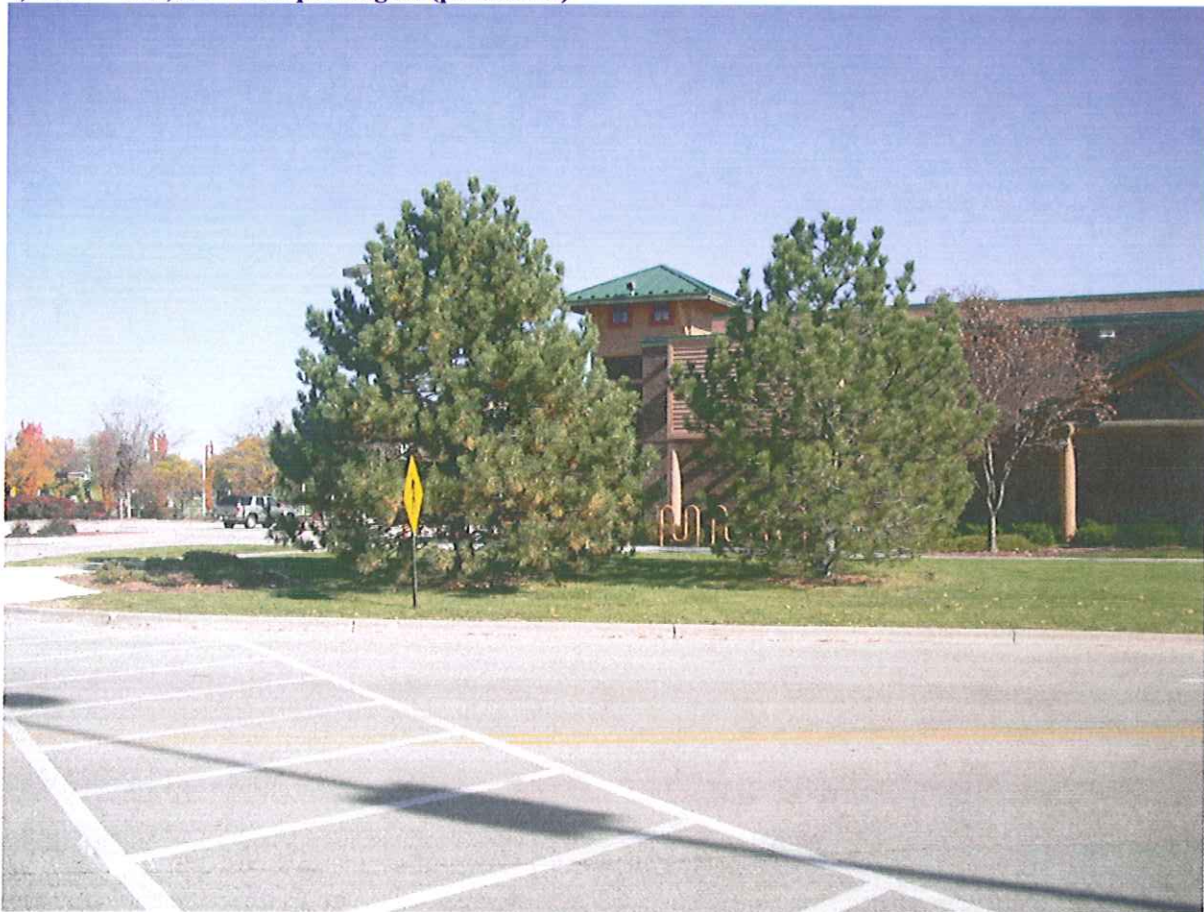
5) View – east, from JCP parking lot (panoramic)
