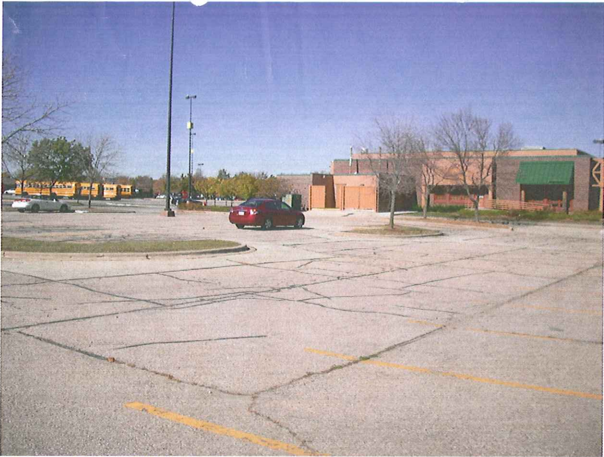
6) View – north, from Mall entrance drive
