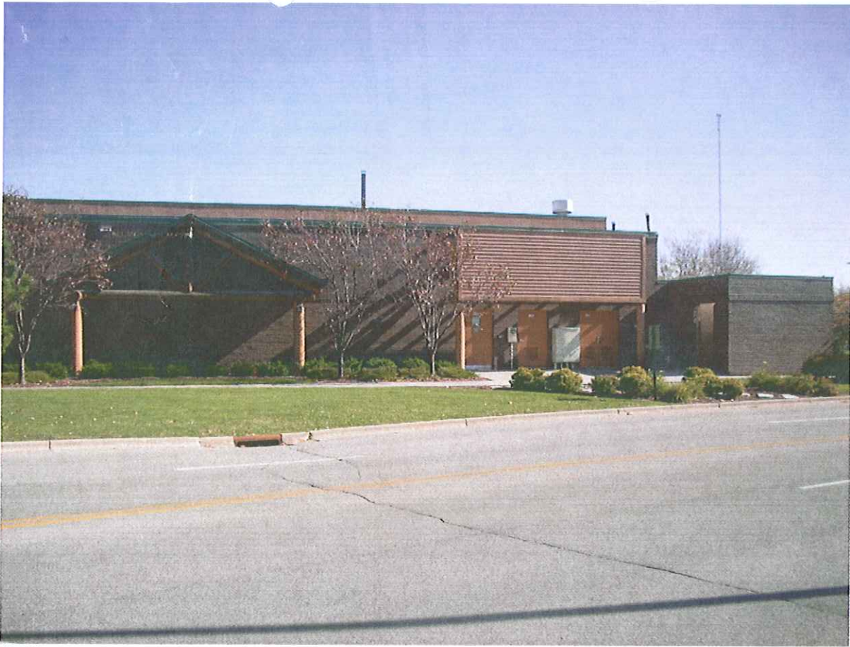
4) View – east, from JCP parking lot (panoramic)
