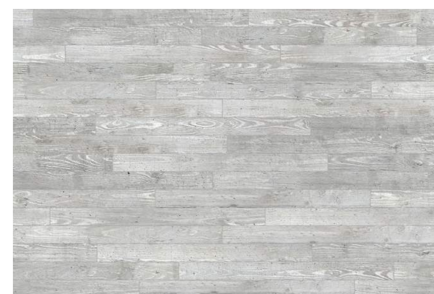
BOARD FORMED CONCRETE
