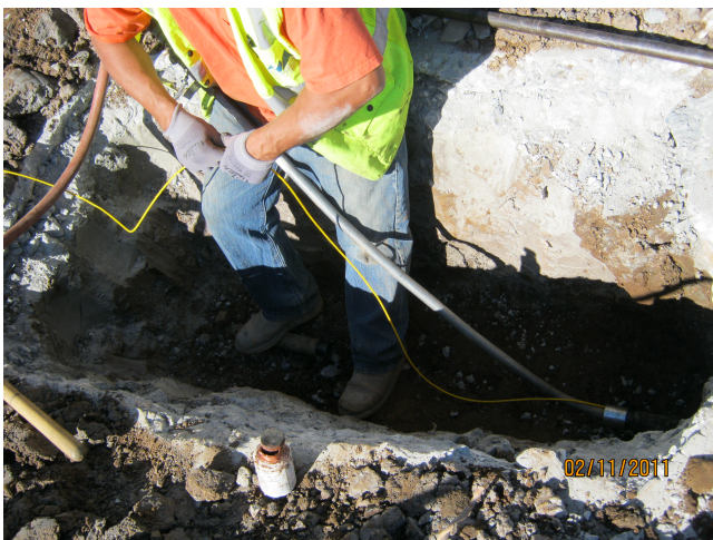
Working with conduit in a trench.
