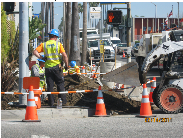
Installing Fiber and Conduit
