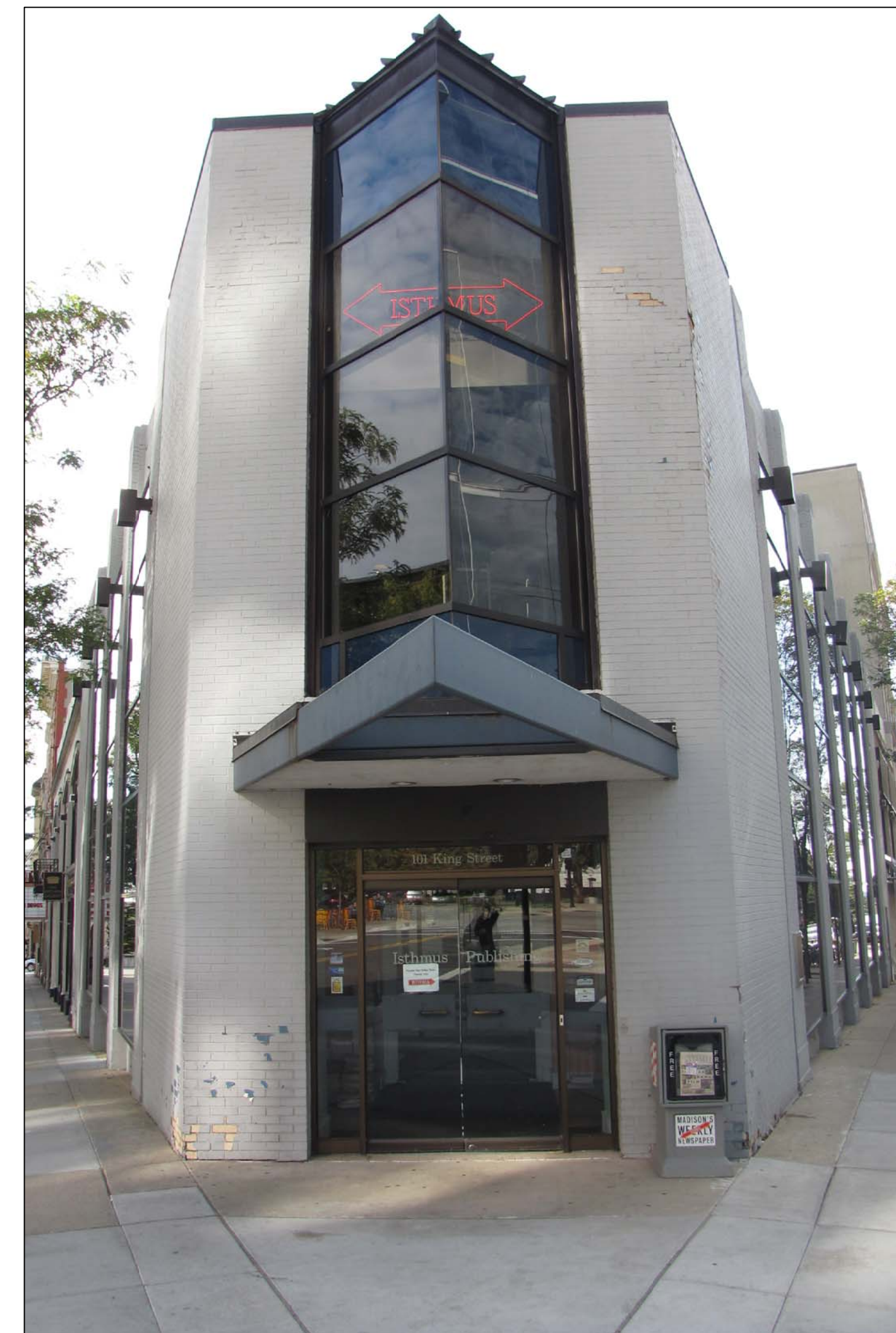
5 VIEW OF MAIN ENTRY NA
