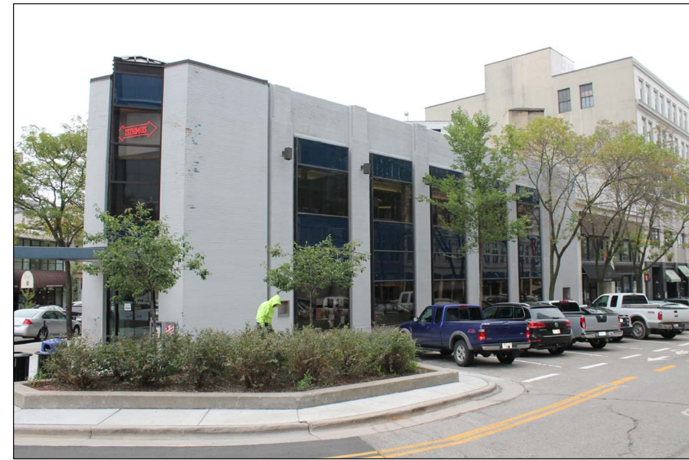
1 VIEW OF PINCKNEY FACADE NA
