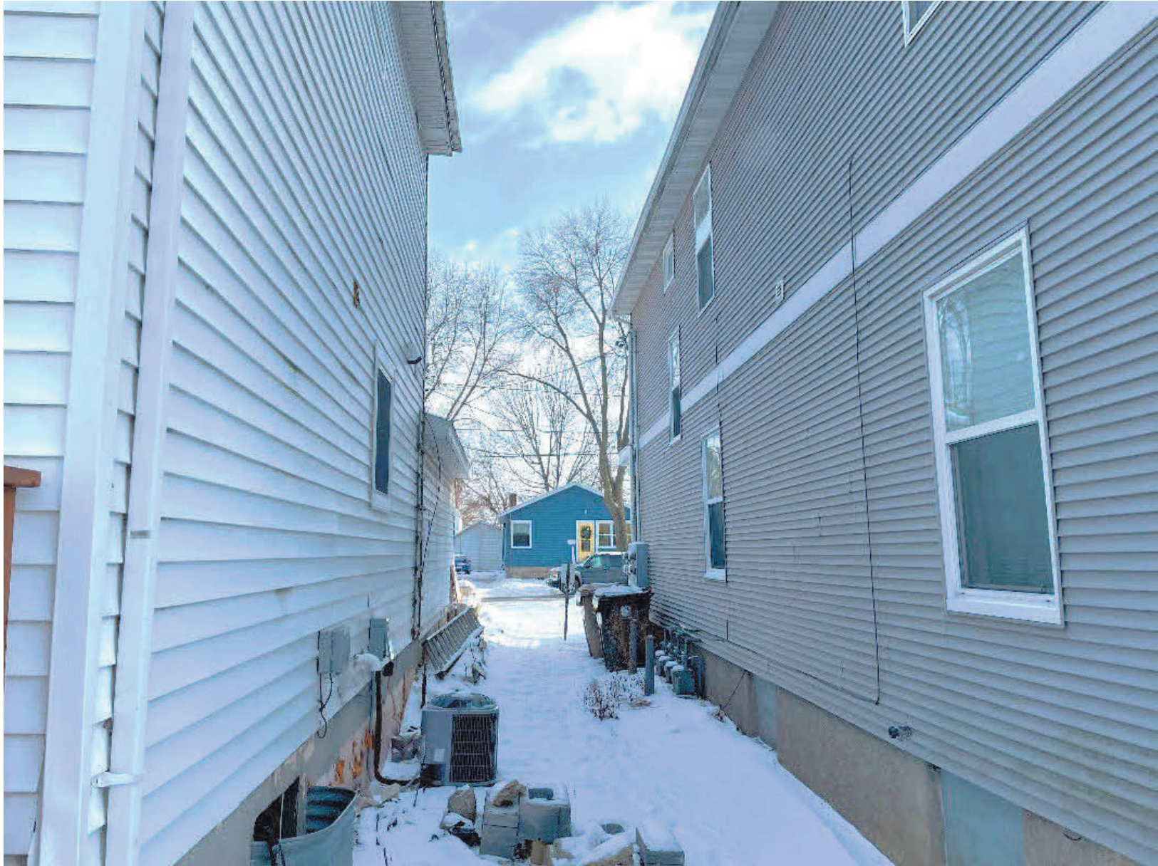
VIEW BETWEEN STRUCTURES, VARIANCE SIDE
