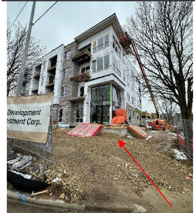
Main Entrance Build Up
