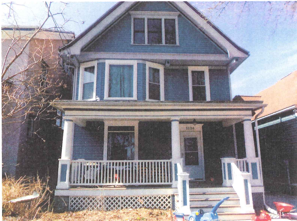
EXISTING FRONT VIEW
