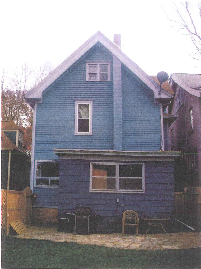
EXISTING REAR VIEW.
