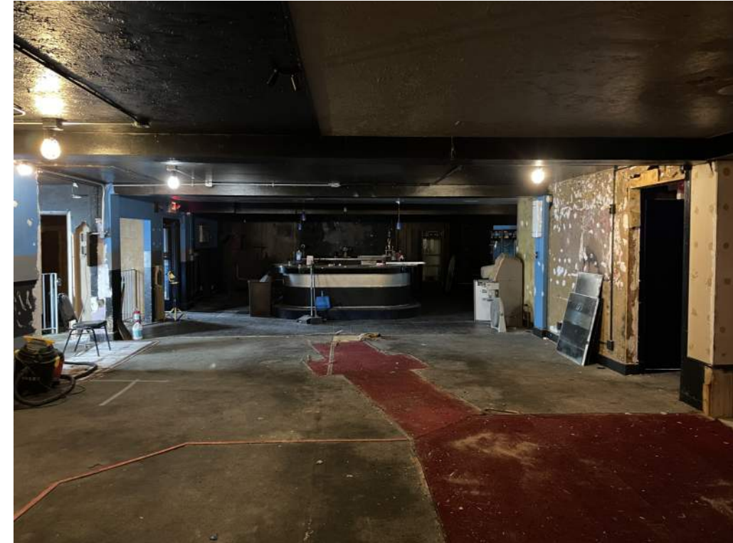
INTERIOR VIEW TOWARDS ENTRY
