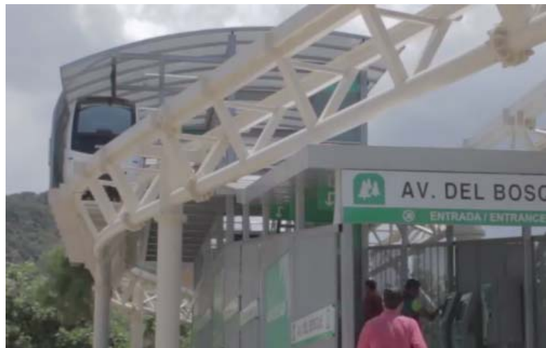
Figure 7 Example of Structure Supporting Pods
