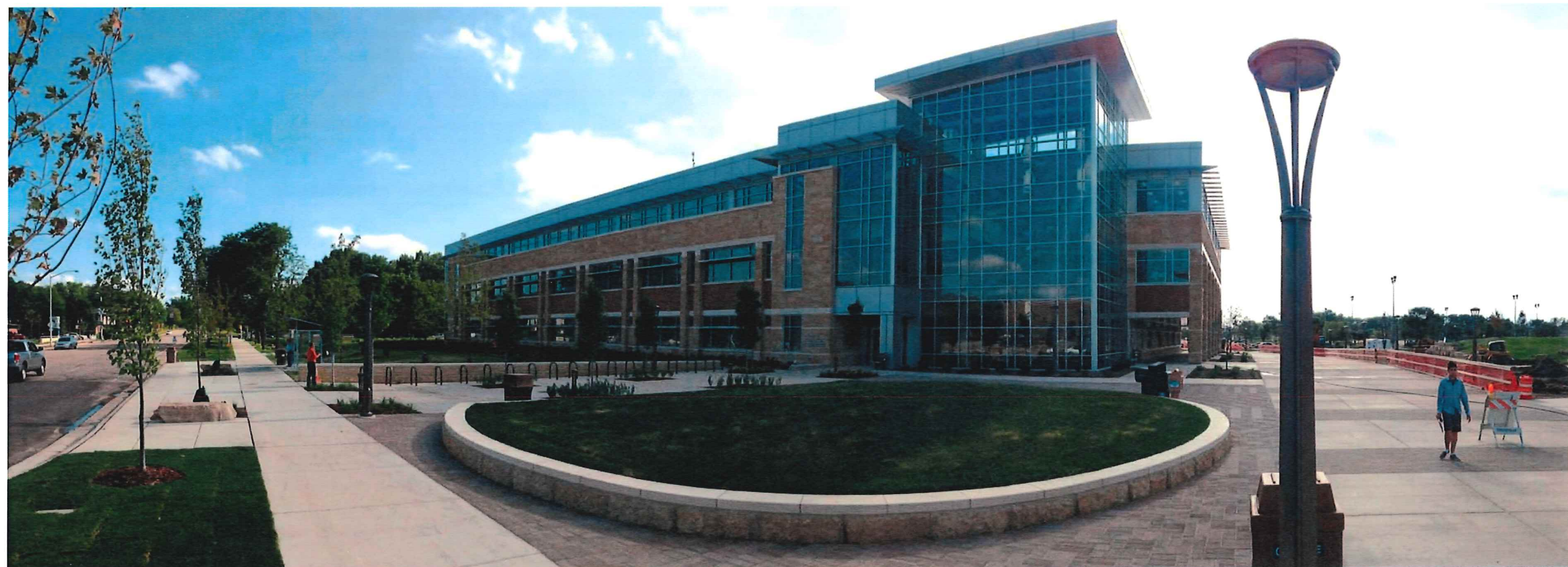
A1: VIEW LOOKING WEST FROM WRIGHT STREET TO HEALTH EDUCATION BUILDING
