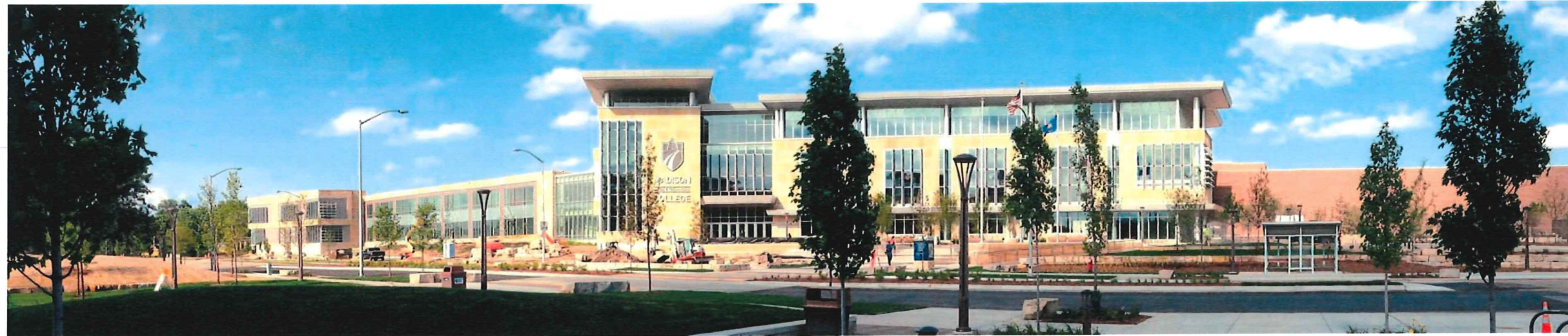
C1: VIEW LOOKING EAST FROM WRIGHT STREET TO THE TRAUX BUILDING/MITBY THEATER/REDSTEN GYMNASIUM
