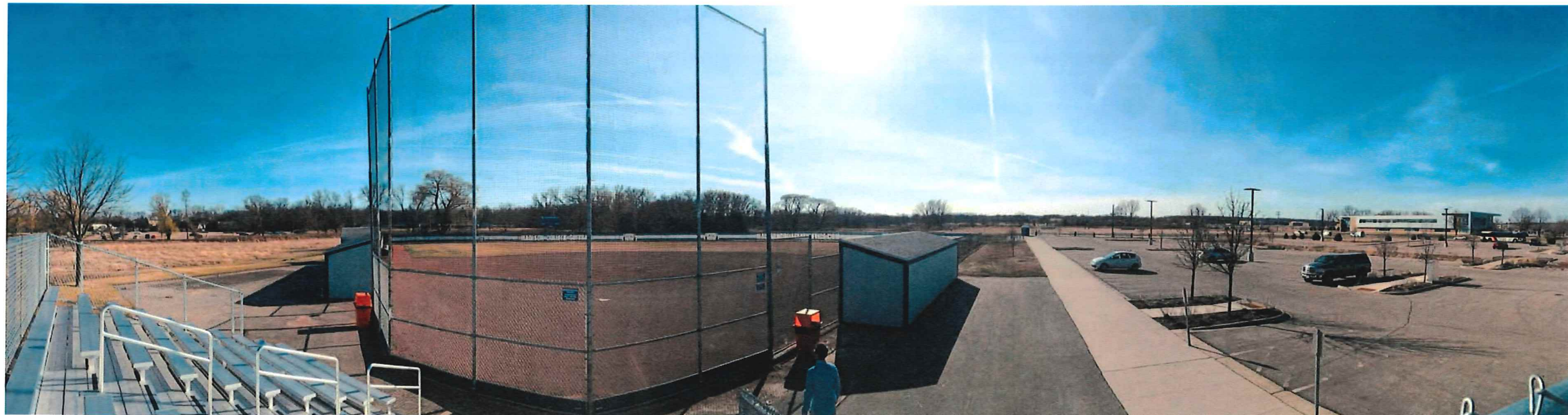
A1: VIEW LOOKING WEST AT THE EXISTING SOFTBALL DIAMOND AND PARKING LOT
