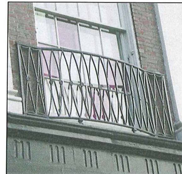
Painted Metal Railing
