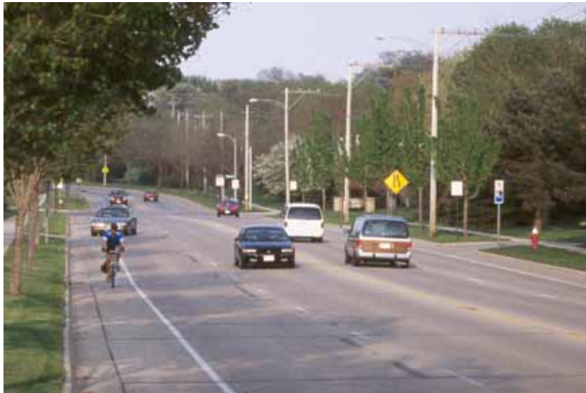
Bike lanes are a typical improvement for arterial streets. Image: Arthur Ross
