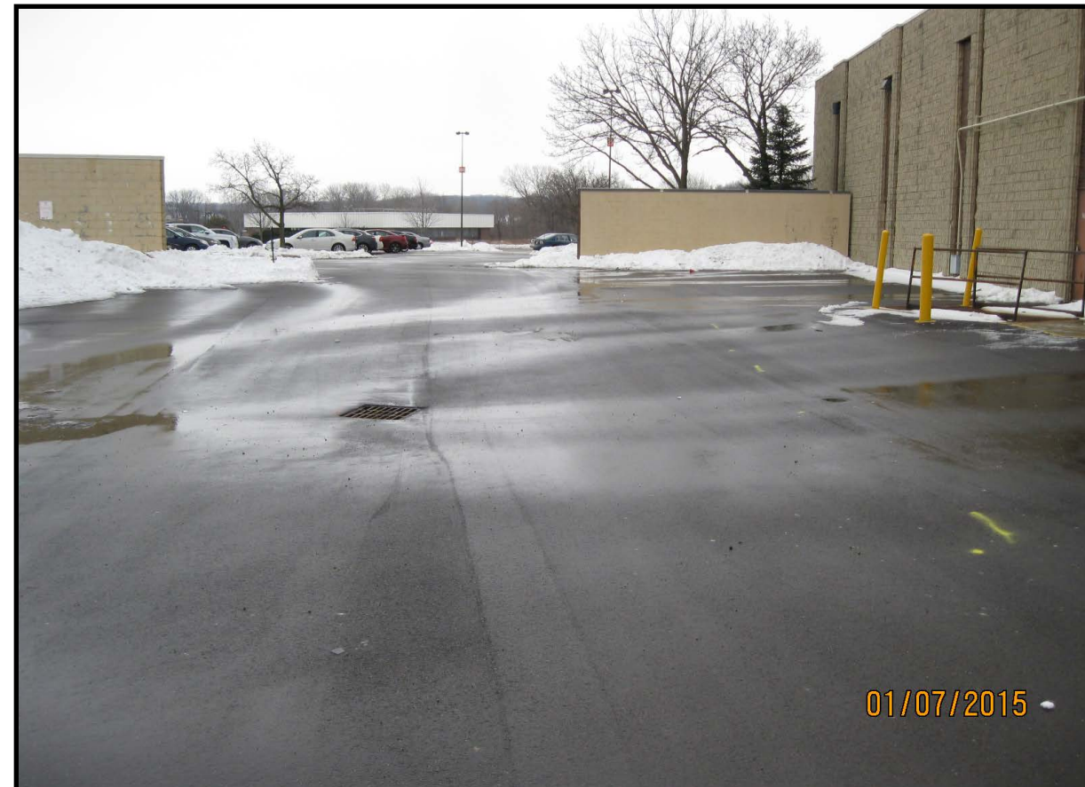
Maintenance Drive between Site and Adjacent Building
