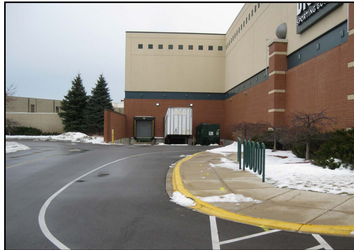
Maintenance Drive Between Site and Adjacent Building
