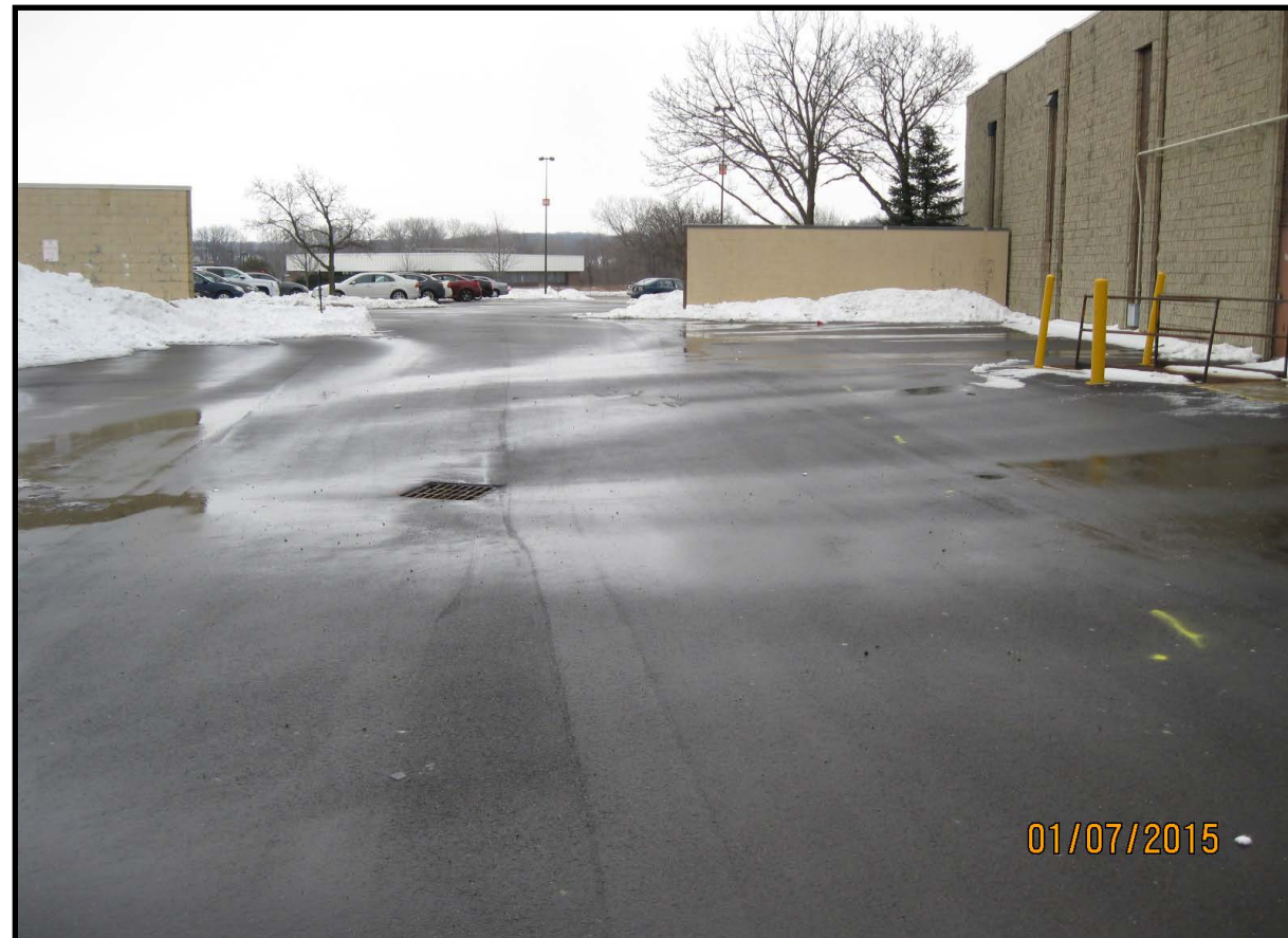
Maintenance Drive between Site and Adjacent Building
