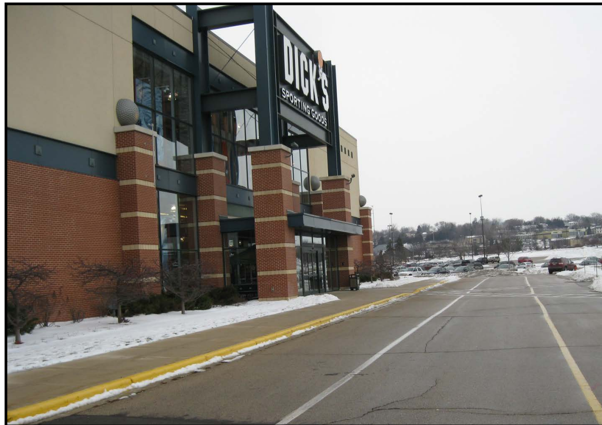
Facade of Adjacent Building to the North
