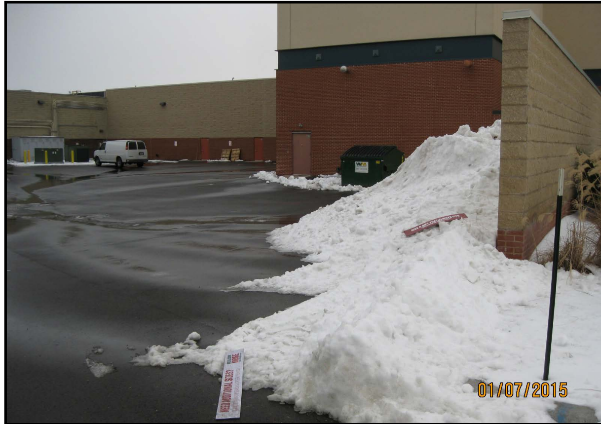
Maintenance Access and Snow Storage
