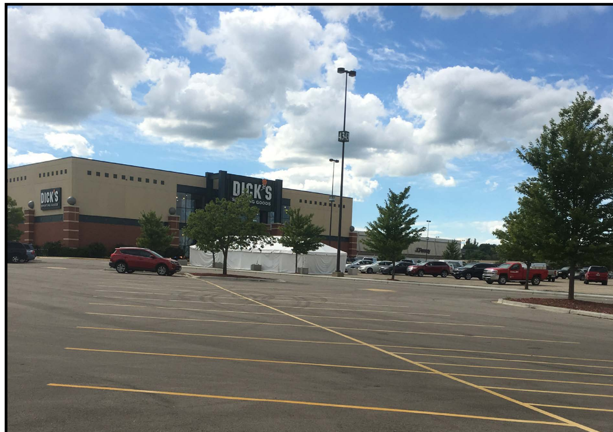
Existing Parking Lot Islands and Landscape
